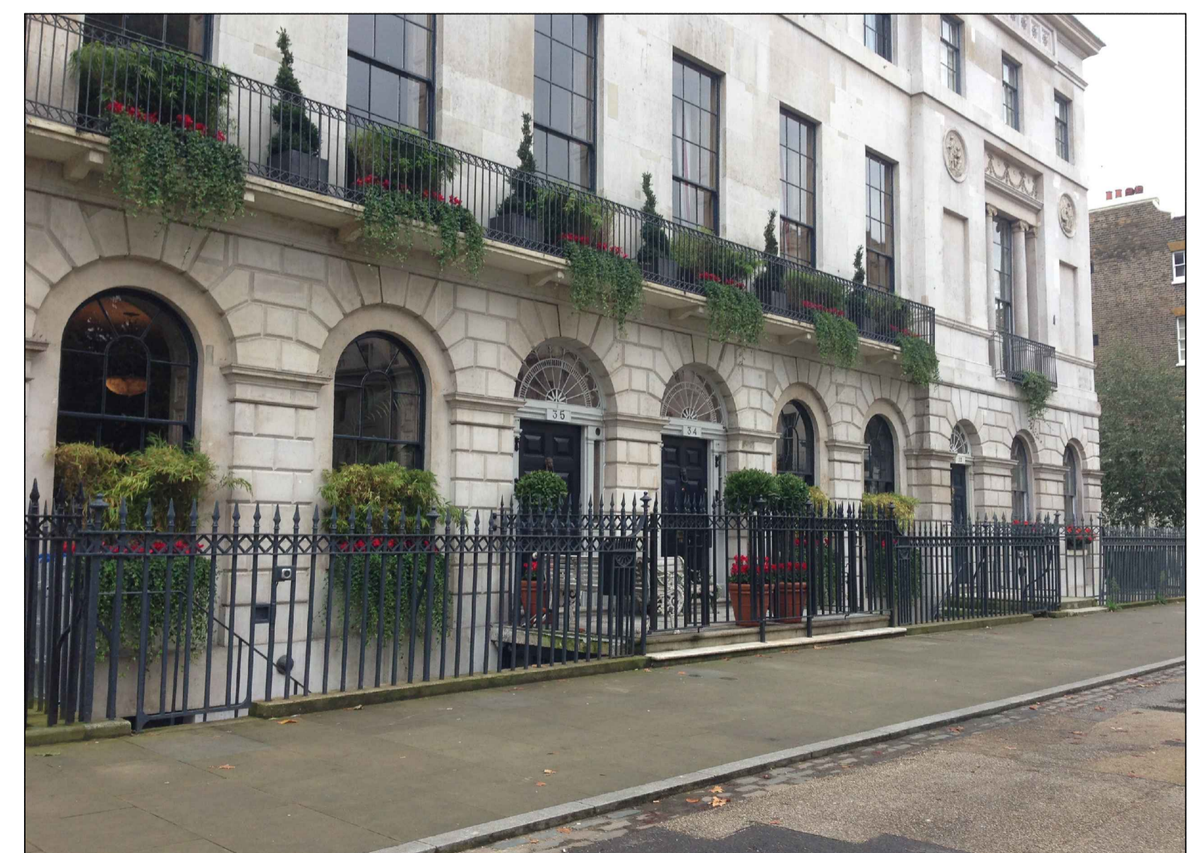
PHOTOGRAPH OF FRONT ELEVATION
