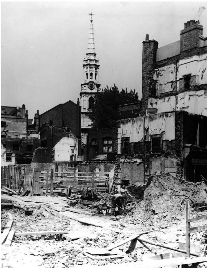
Further clearance work of the Stacey street bombsite, c. 1941
