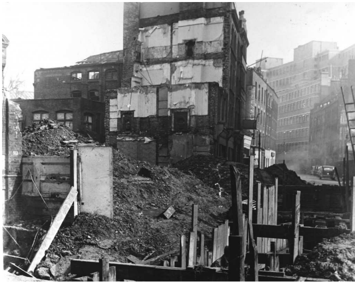
Looking west up New Compton Street, dated 3 rd September 1941
