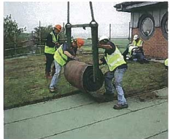
▲ Long length rolls being craned into position and installed.
