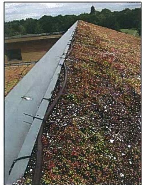
Sedum blanket being applied to a steep sloped roof, fitted with both retention strips and drip line irrigation.
