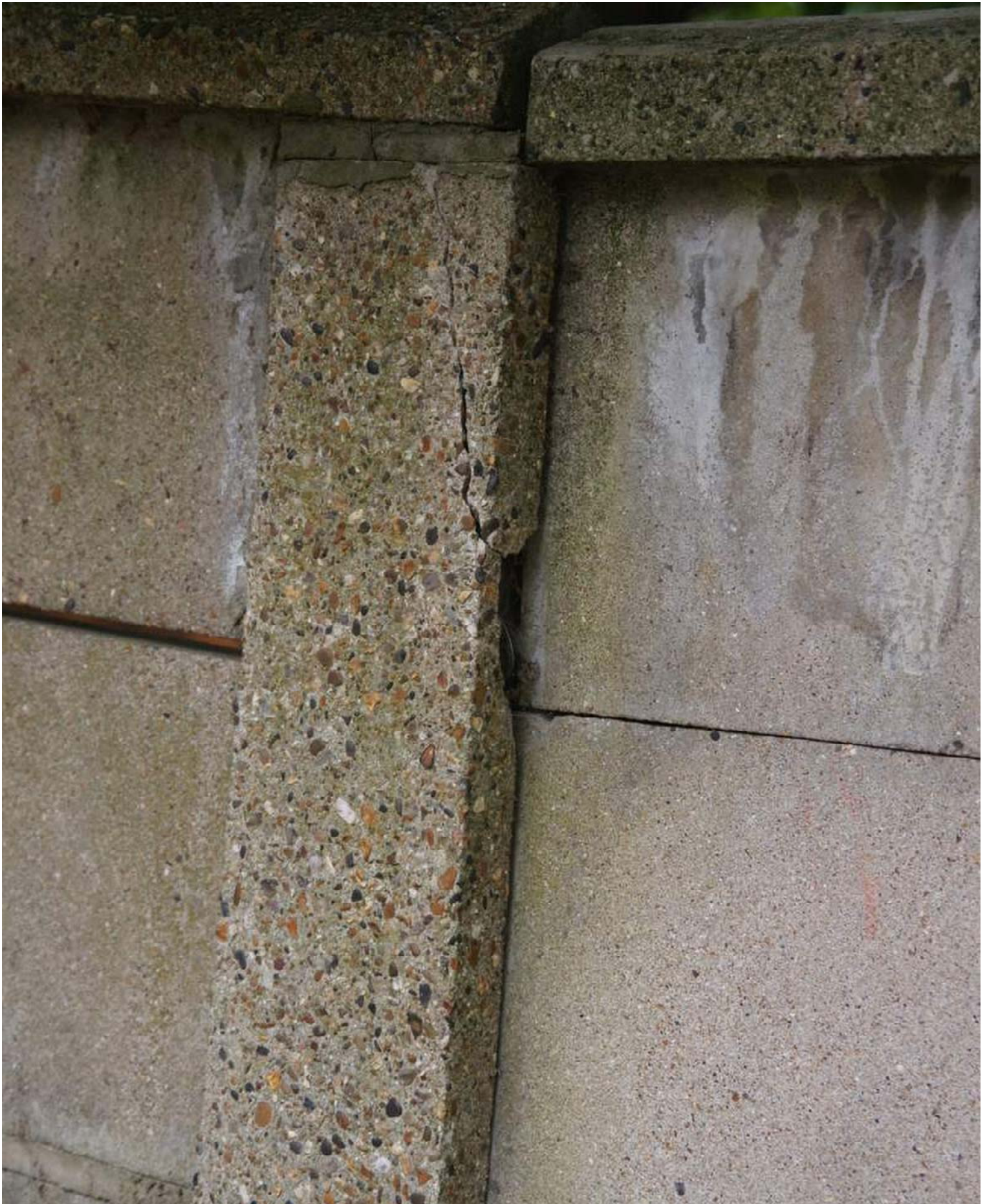
Photo 22 - Detail of existing concrete post top
