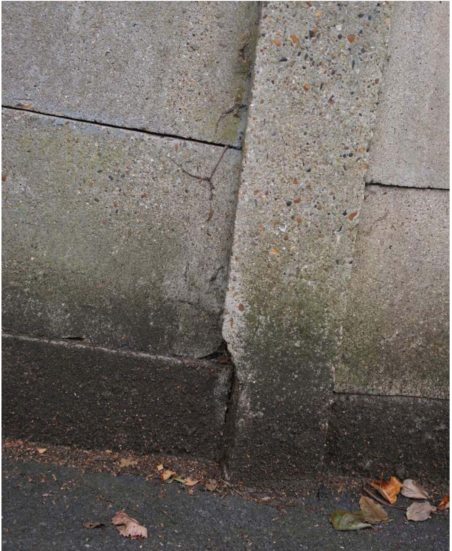
Photo 21 - Detail of existing concrete post bottom
