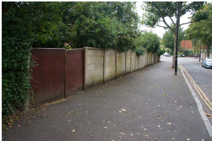
Pavement on St Albans Rd, adjacent to 34 Brookfield
