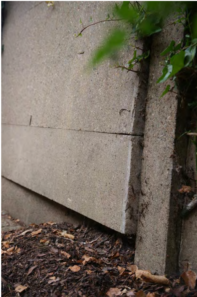
Panels on the fifth section of wall clear out of slotted post
