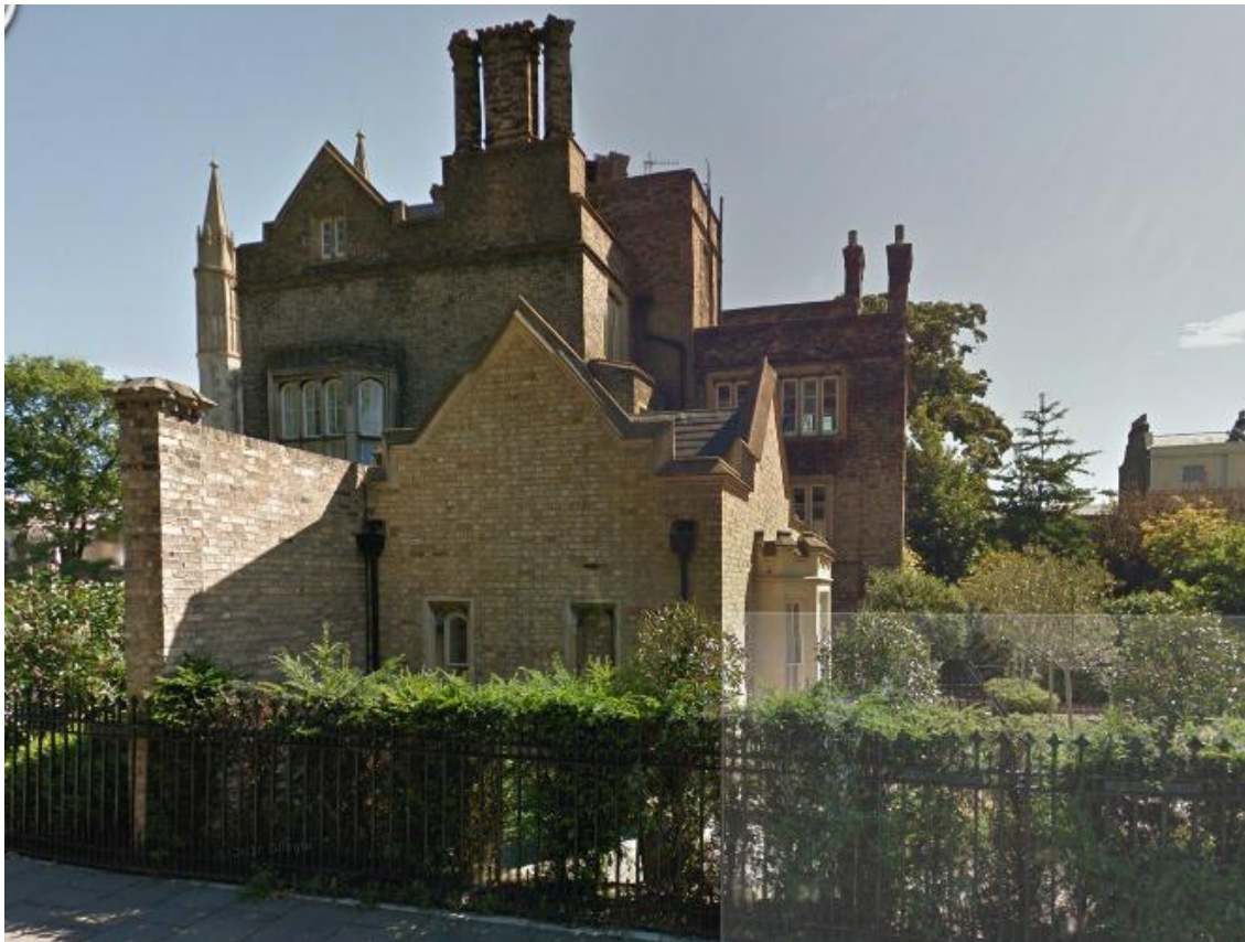
1.6 Side of property
