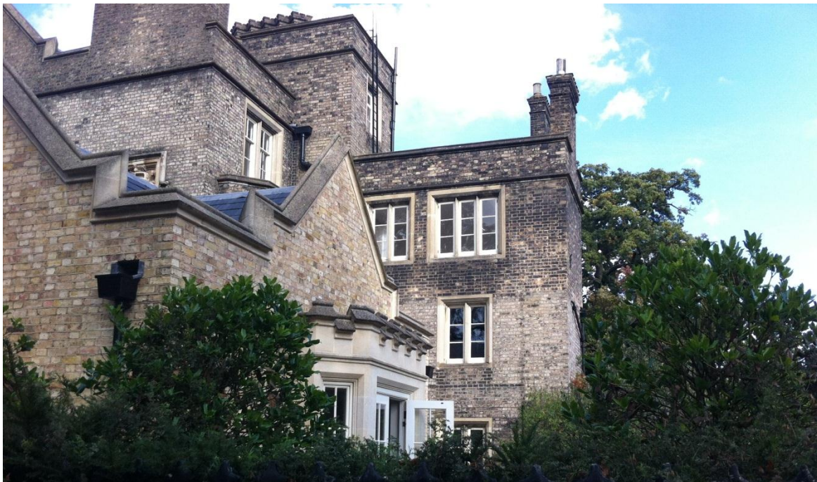
1.2 Rear of property where new window will be placed.
