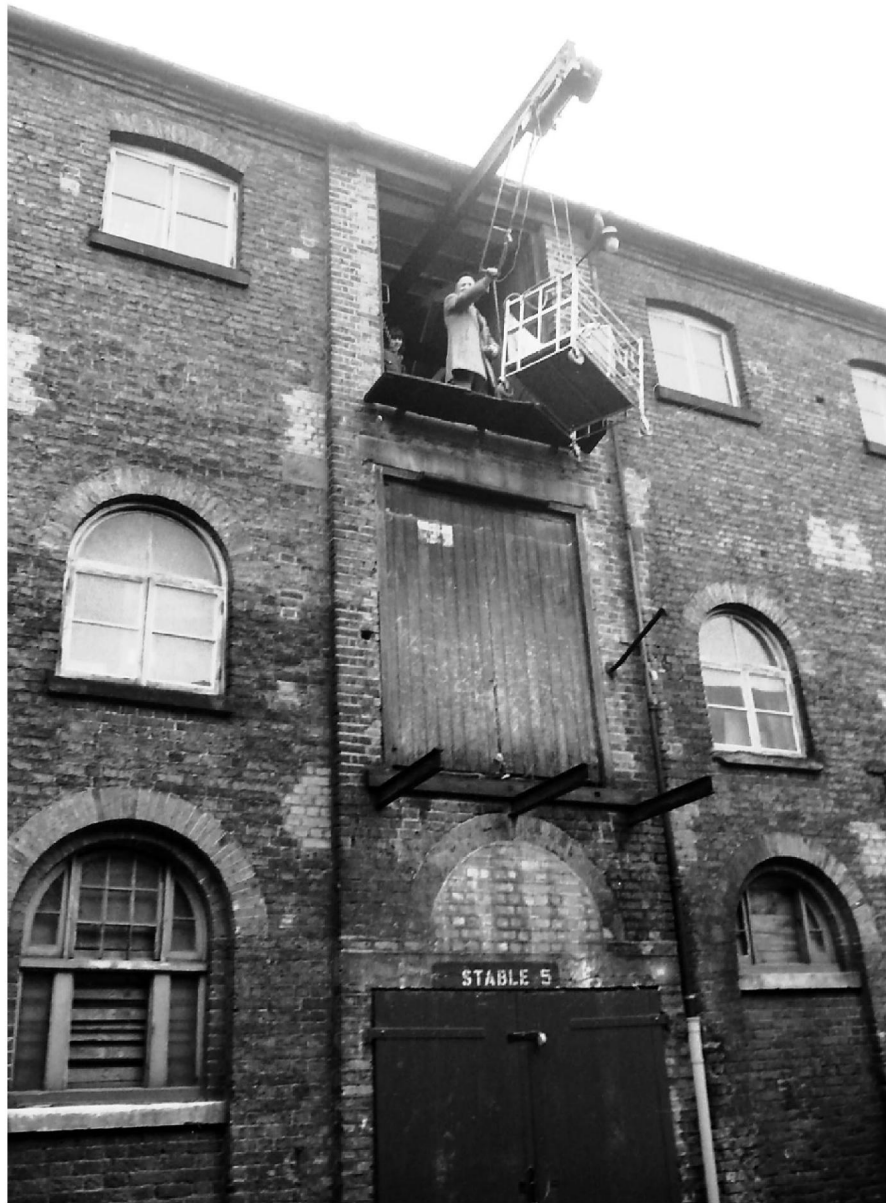
Section 5, 22 Feb 1975 (MTT510_5A). The loading doors here are seen to have been widened under concrete lintels during the 20th c. Note functional hinged flap at second floor. Doors fitted at first floor are less recessed than traditional doors.
