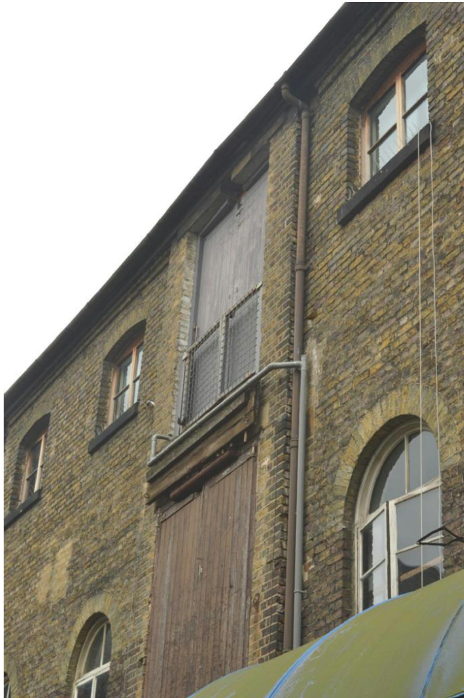
Section 5 today. Note the widened first floor doors have been replaced since 1975 and are now completely flush.
