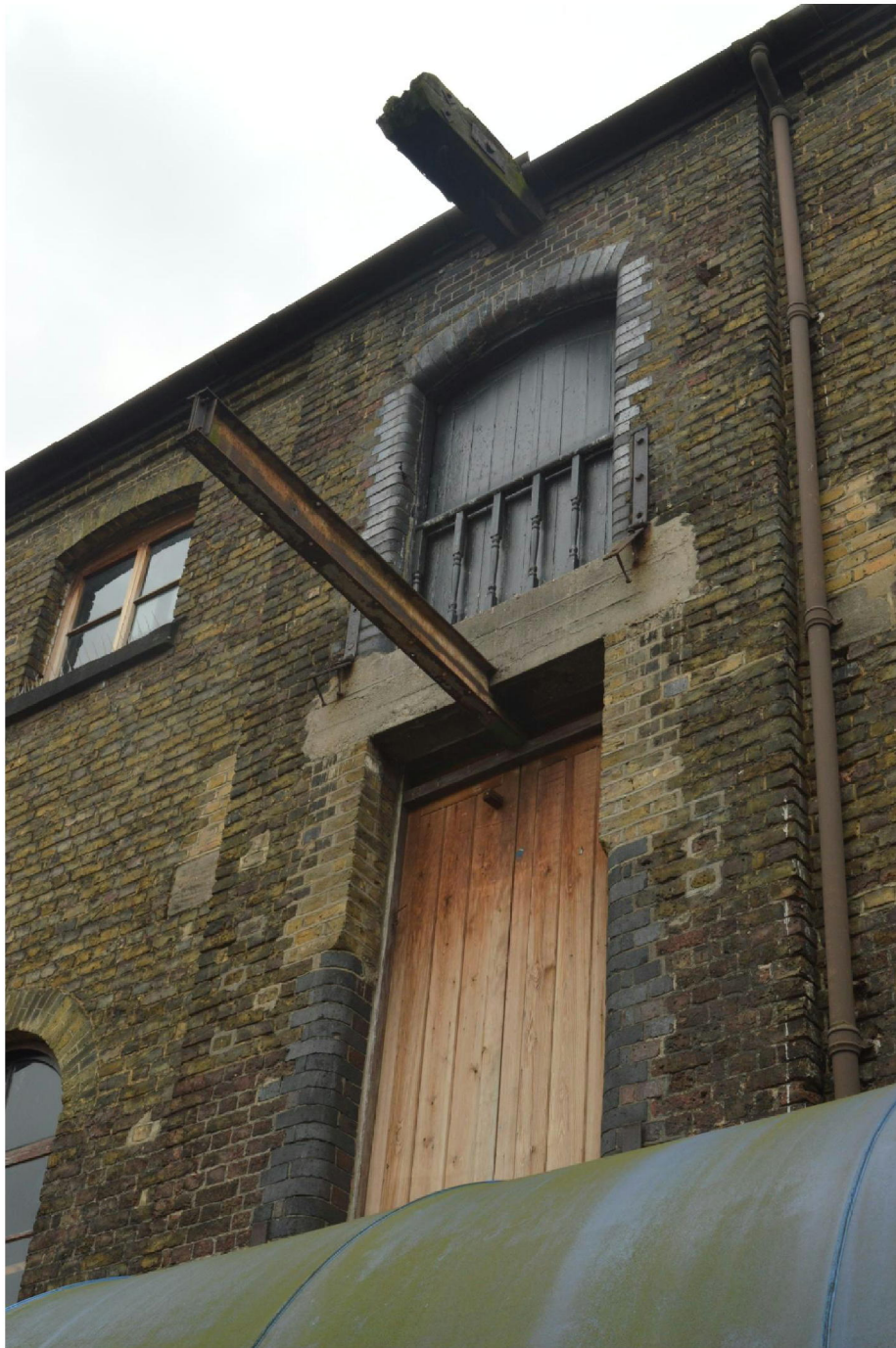
Section 4 today. Note original timber cathead beam and blue brick reveals to these loading doors
