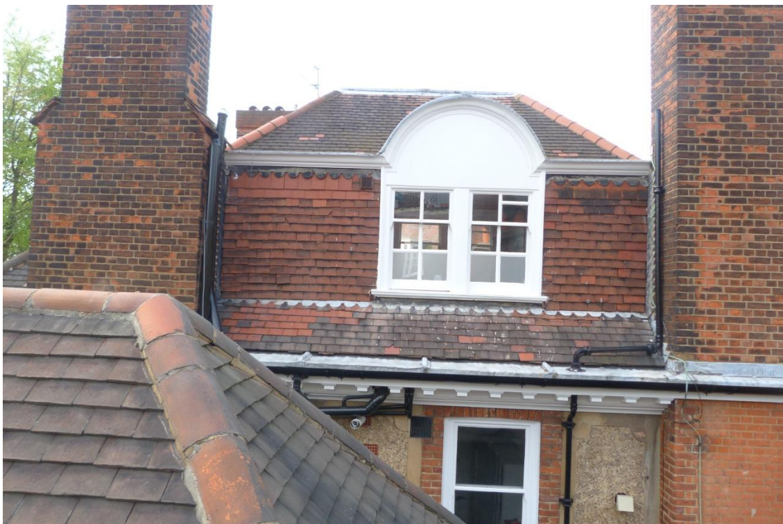
Neighbouring dormer (higher than existing ridge)
