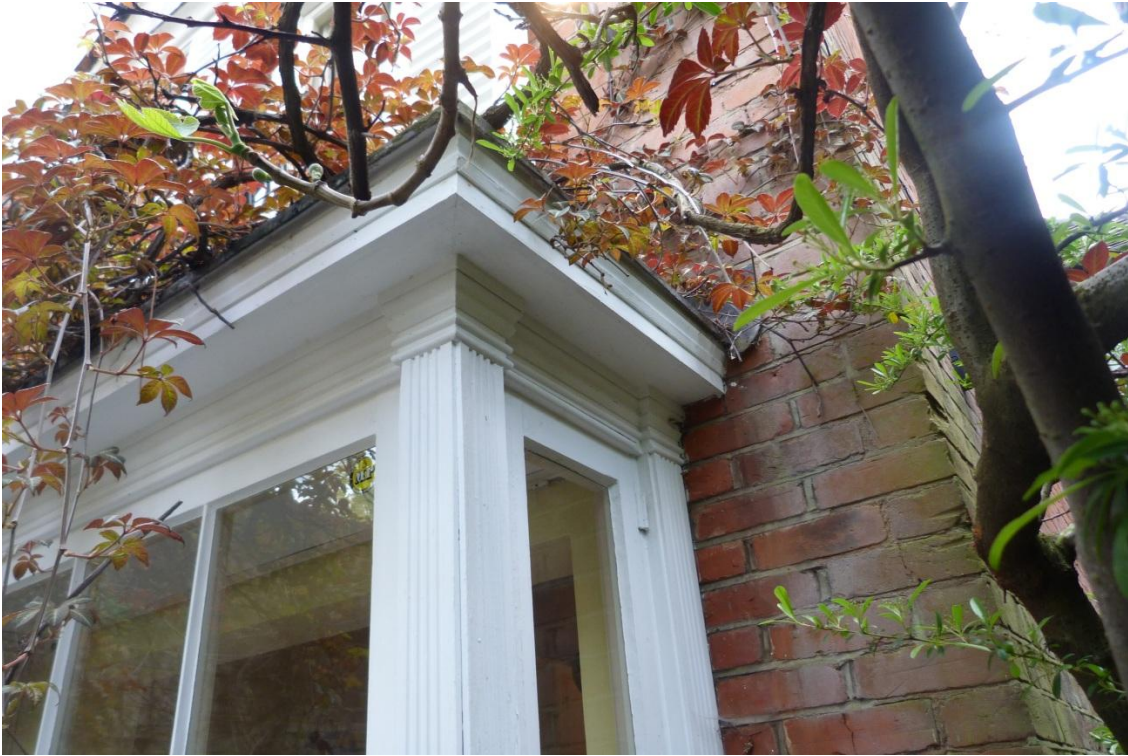
Protrusion of Bay
