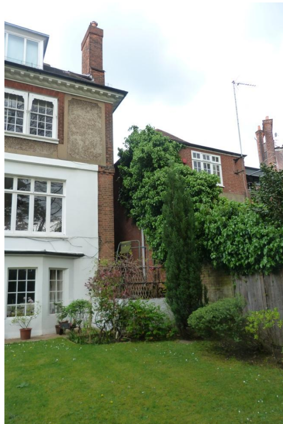
Rear aspect showing the relationship to neighbouring property
