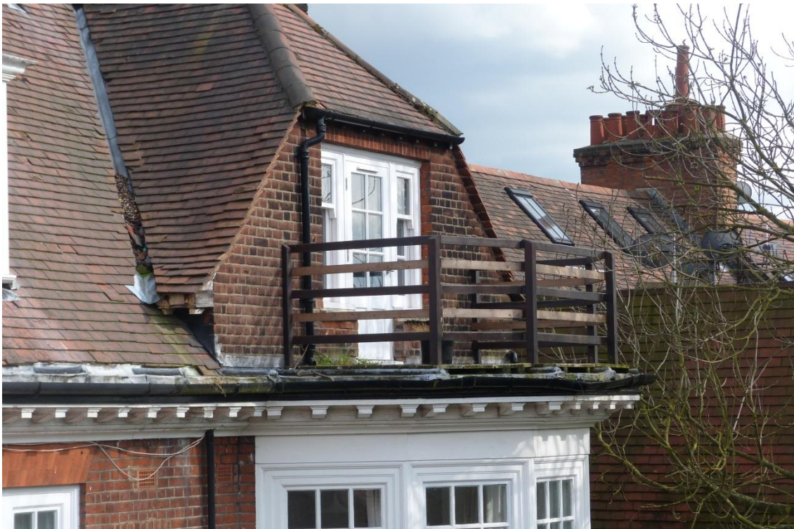
Balcony of neighbouring dwelling
