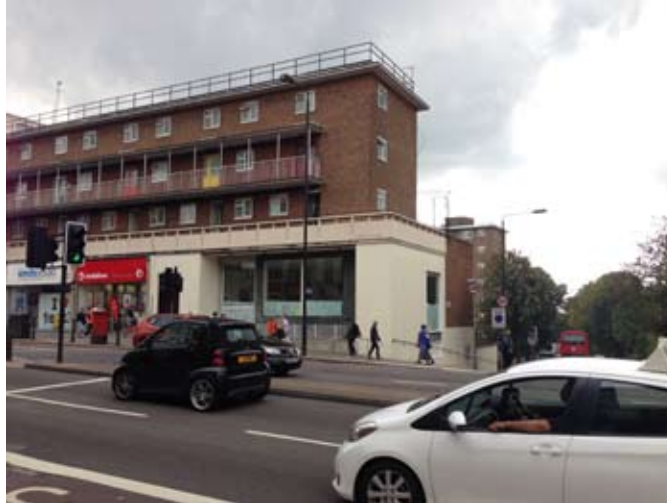
View from north east
