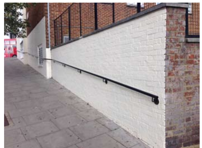
Pavement on Fairfax Road, Finchley Road at top
