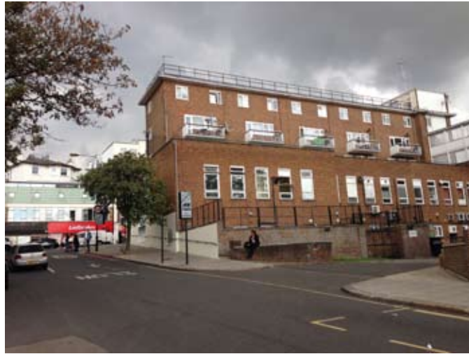
View from Fairfax Road, service road to right
