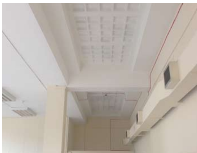
Painted out skylights onto flats gallery over
