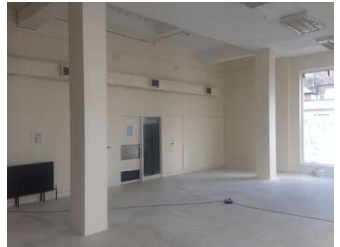
View north west
