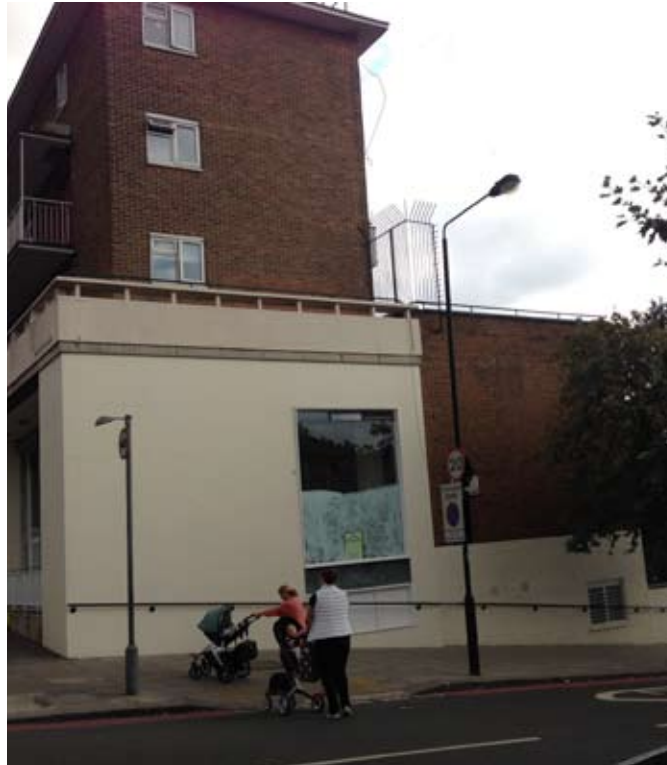
Side view along Fairfax Road
