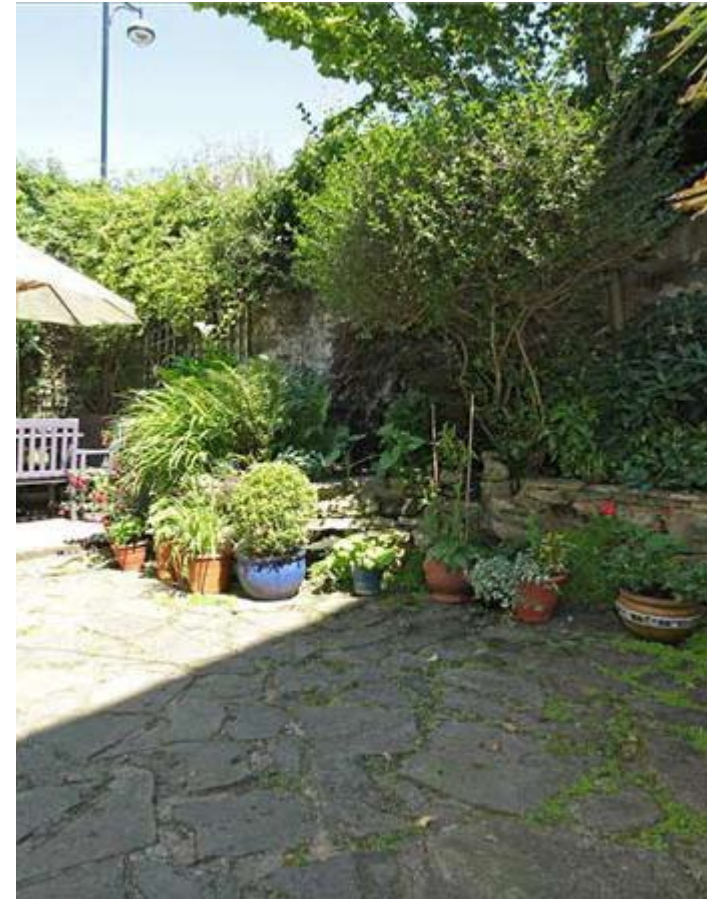
Transforming the yard with new surface and planting
