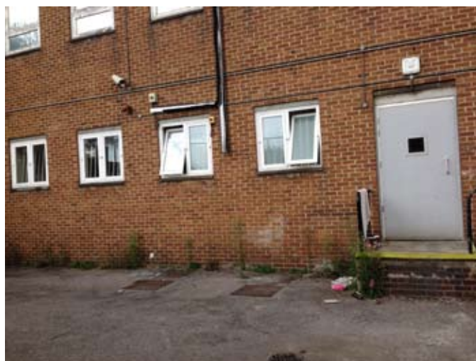
View of basement door and windows within service yard
