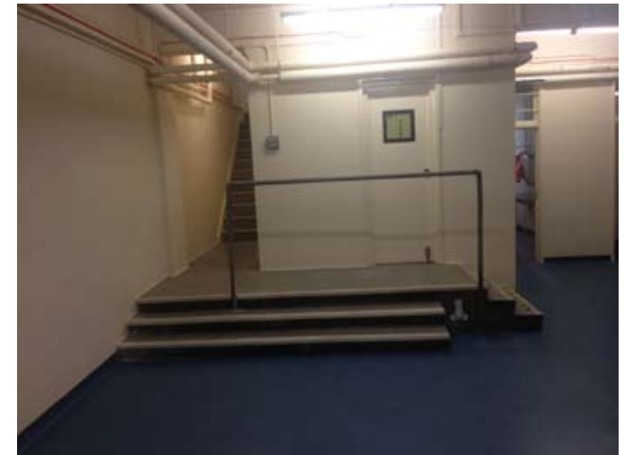
Landing and stair to ground floor
