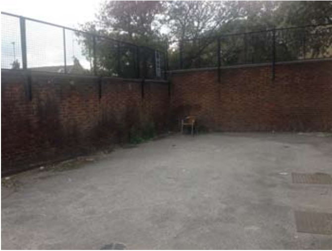
View north west
