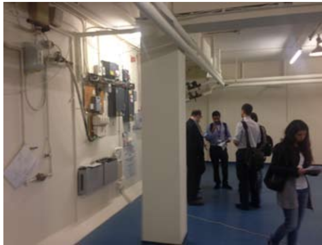
Front wall below Finchley Road
