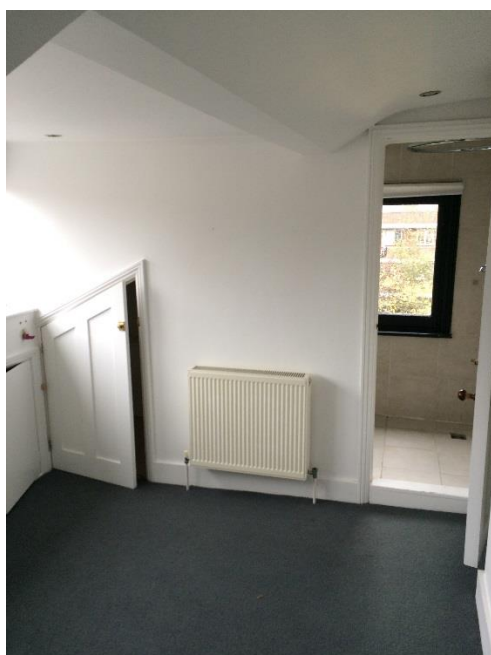
Existing en-suite to second floor rear bedroom to be refurbished
