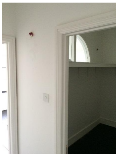
Modern partitioning within master bedroom to be removed
