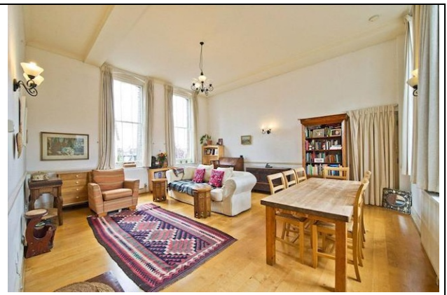
View of 'existing' Reception / Dining Room. Note - new flooring and skirtings. Note ceiling is plain with no ceiling roses etc.
