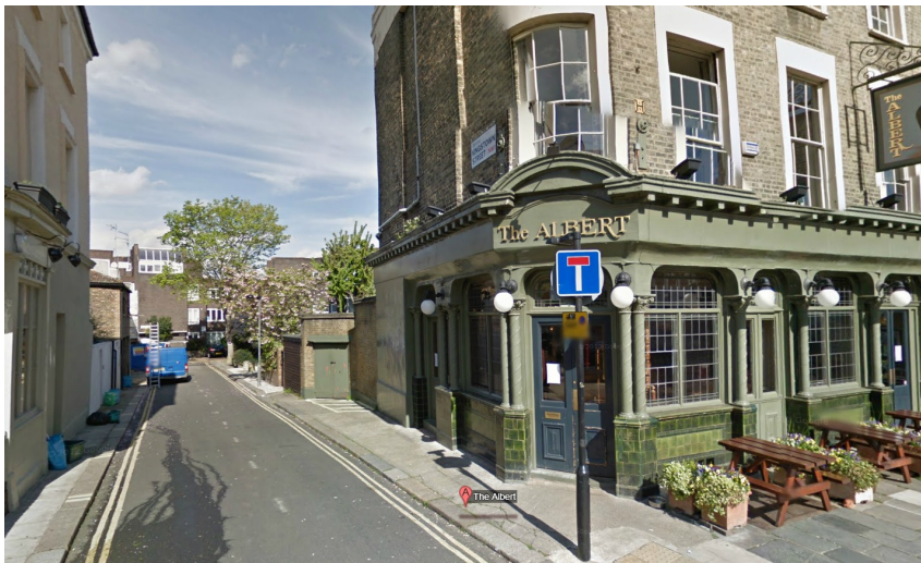
Albert Pub: Photograph facing west down Kingstown Street showing the existing wall and garage behind which the pub garden is located.
