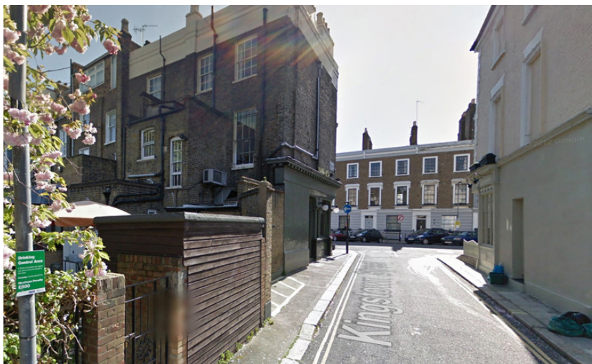
Albert Pub: Photograph facing east along Kingstown Street showing the existing wall and garage frontage onto Kingstown Street.
