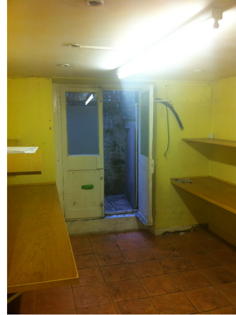
Existing rear elevation lightwell
