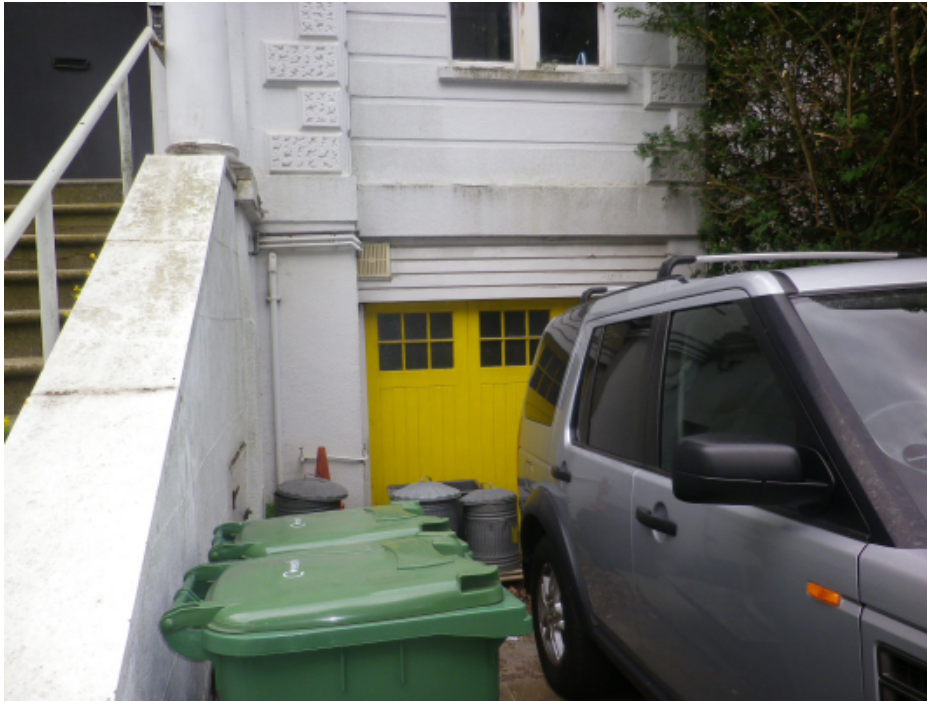
Photo 1 – Front elevation showing garage and parking.
