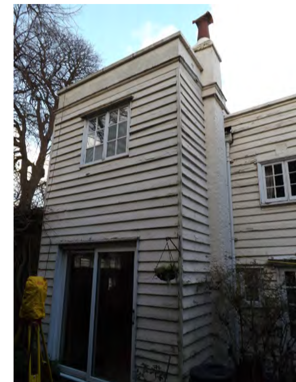
Photograph of rear timber weatherboarding
