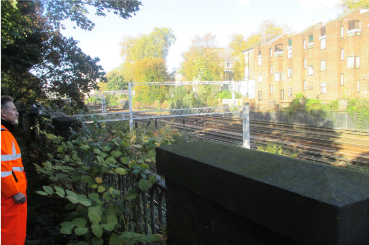
1.1 The site runs along a railway line
