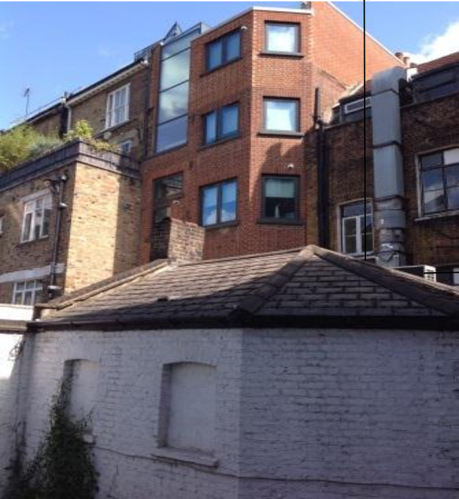
Photo 3- AC unit to be lowered in height and AC unit on flat roof of outbuilding
