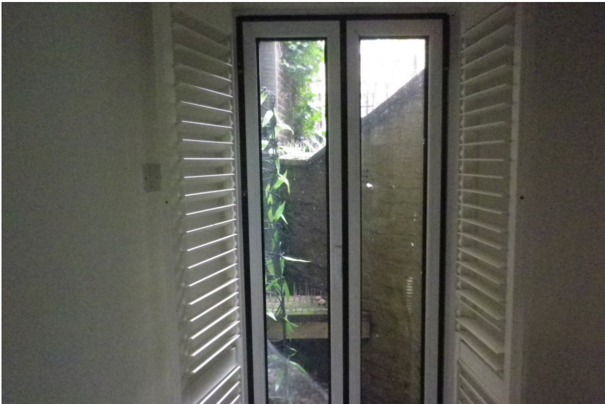
View of & from existing 1 st floor terrace
