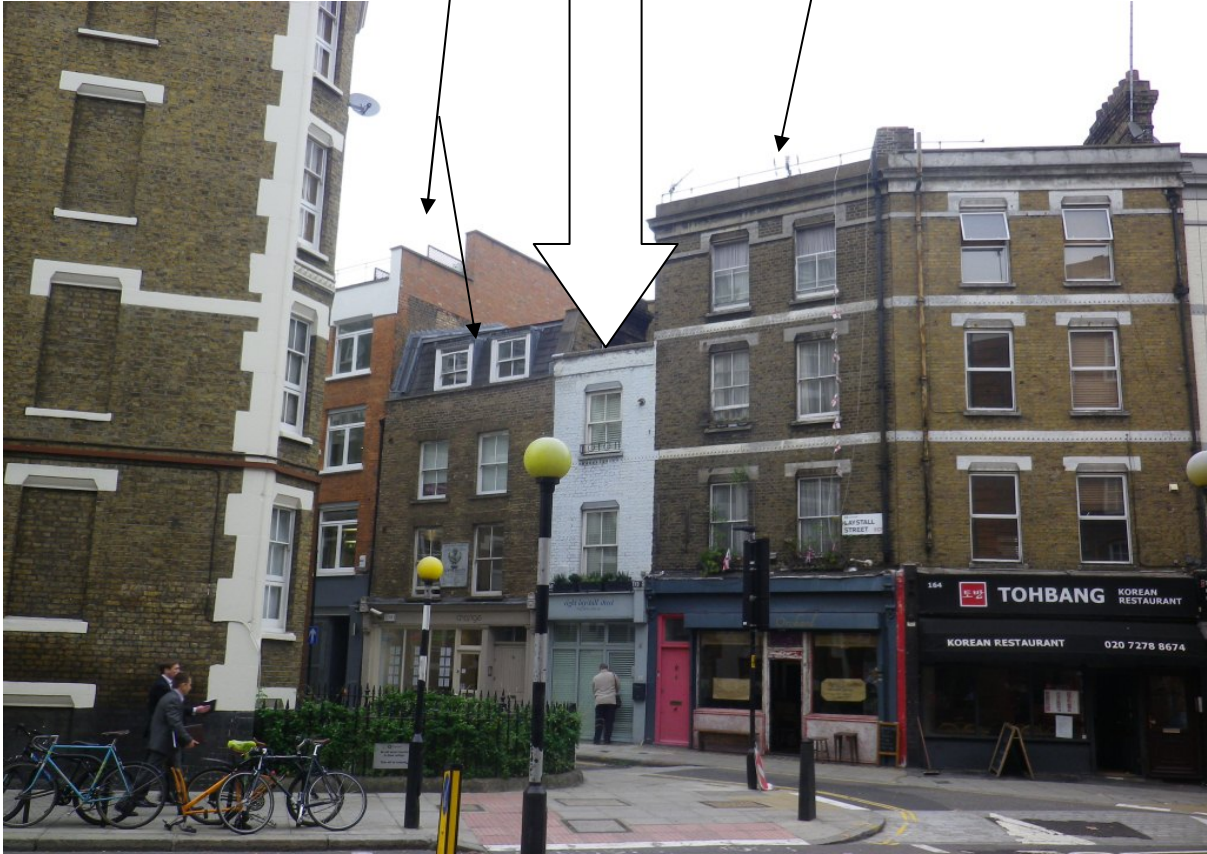
View – front nos. 6, 8, & 10-12 Laystall Street
