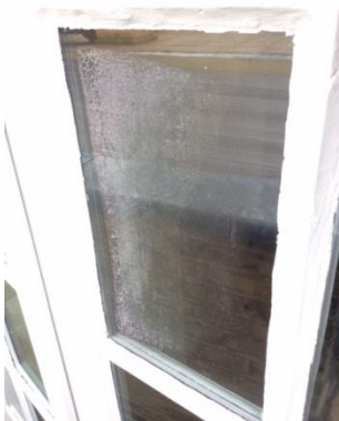
Water moisture between double glazing glass causing cold room
