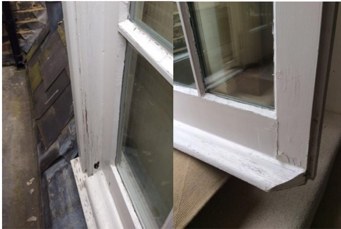
Paint damage and rot allowing water ingress
