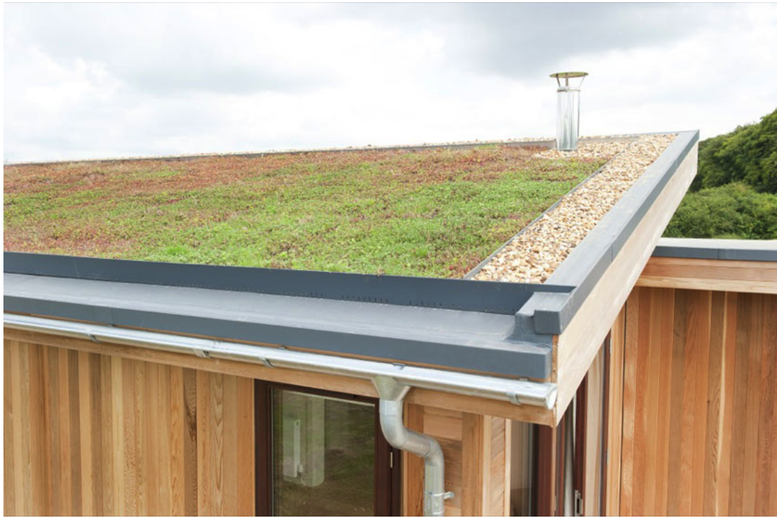
UPSTAND DETAIL TO INSULATED PARAPET WALL WITH METAL CAPPING / AL40 EDGE RETENTION/DRAINAGE TRIM OPTION
