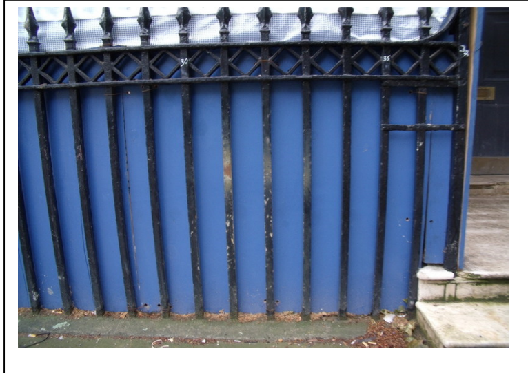
5. Front Railing Palings 31- 36, Corner Support Post 37.
