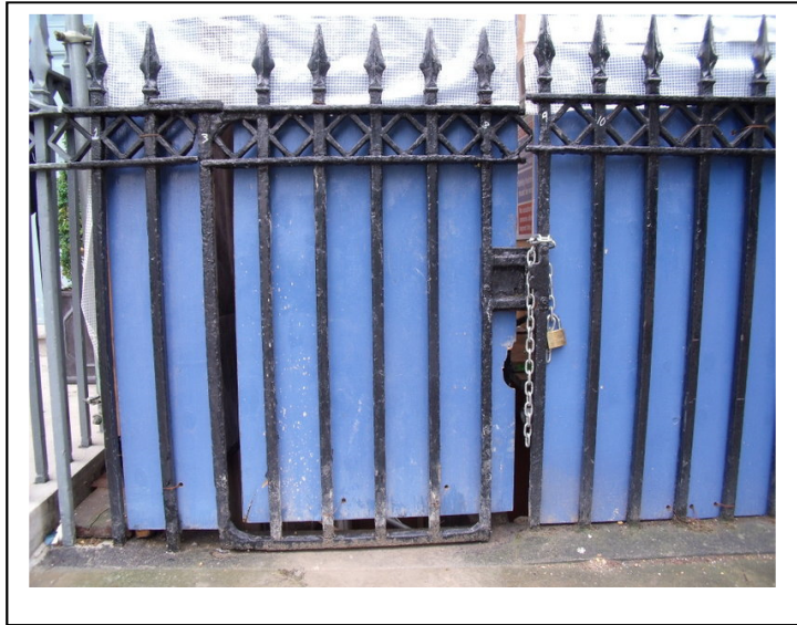
2. Front Railing – Gate Palings 4, 5, 6, 7, 8, Right Hand Side Stile 9
