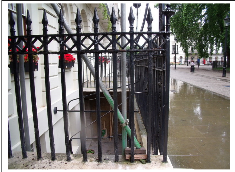
7. Railing at right hand side of front entrance palings 49 – 58.
