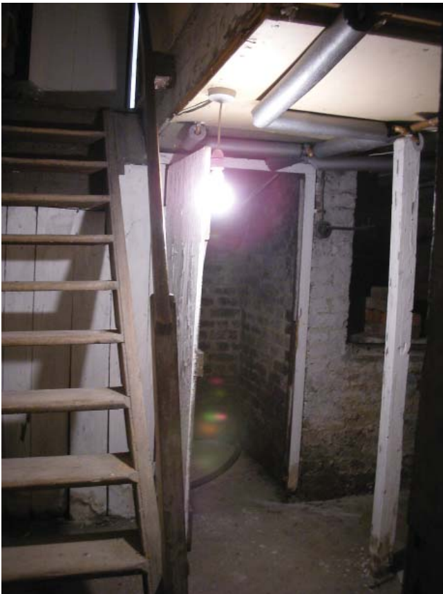
Existing basement access
