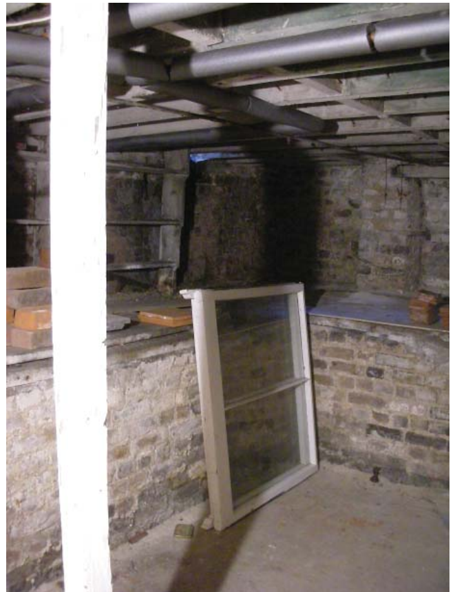
Existing basement area
