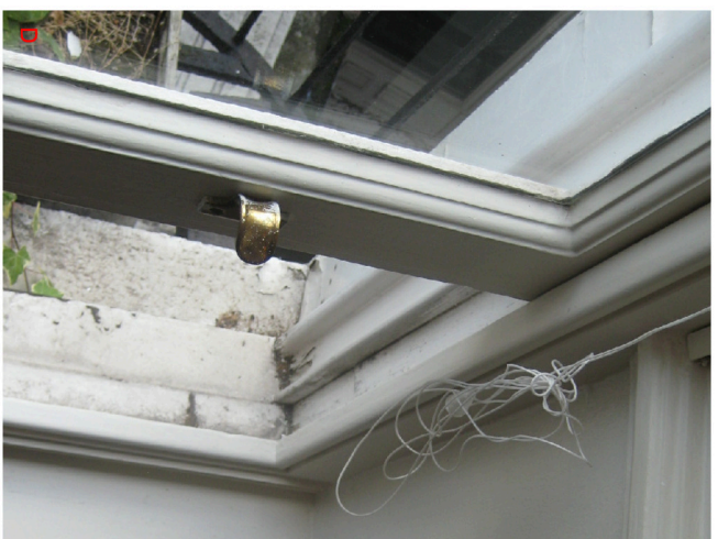
D Photographs displaying typical existing first storey window ironmongery. To be retained
