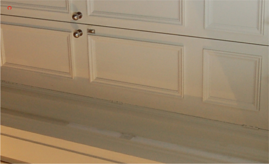
photographs displaying typical existing door handles -First floor stair landing
