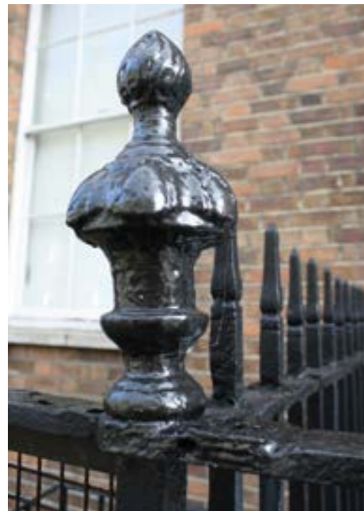
2 - Detail of existing railings
