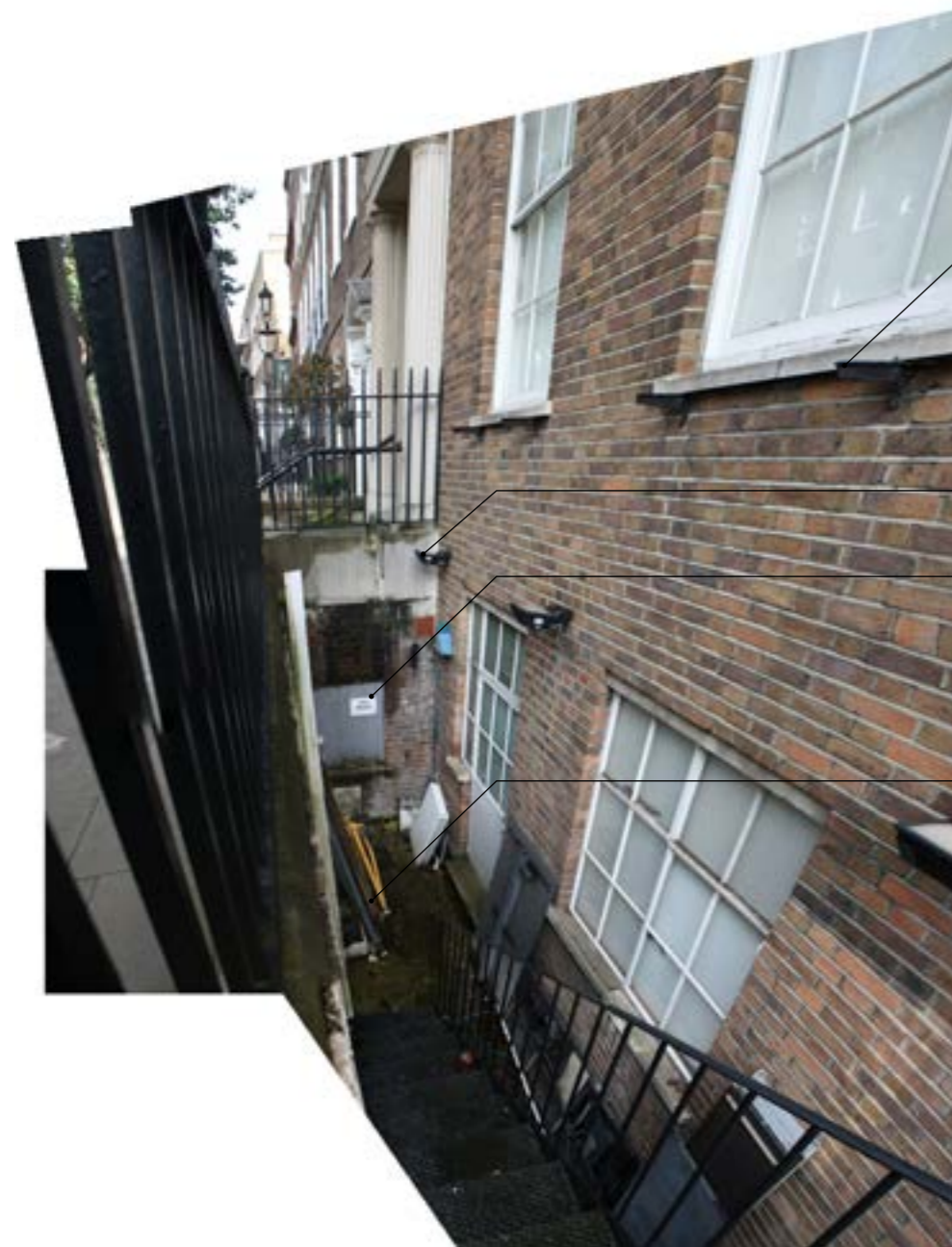
1 - Photo of front lightwell
