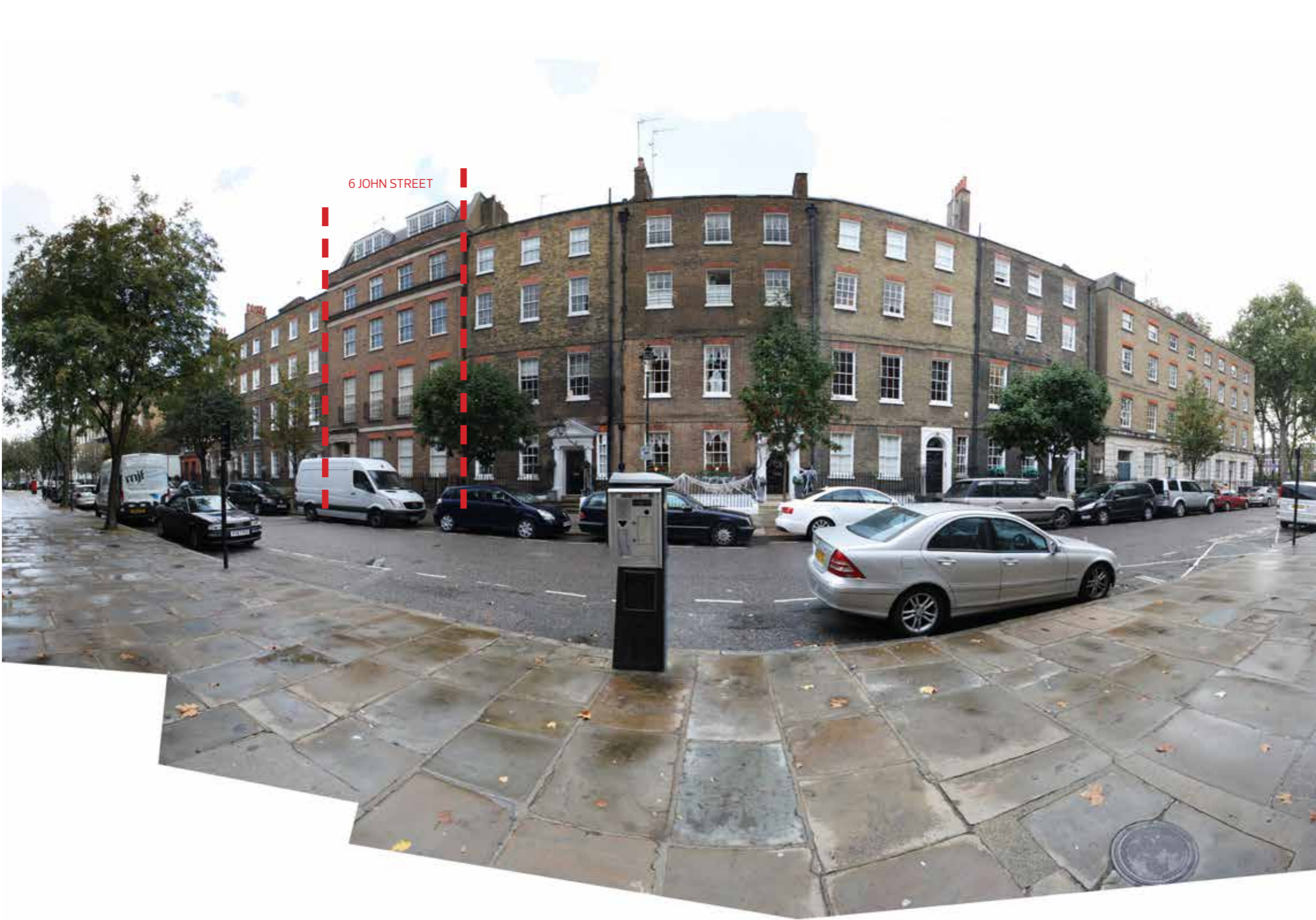
PANORAMIC STREETScape VIEW FROM JOHN STREET
