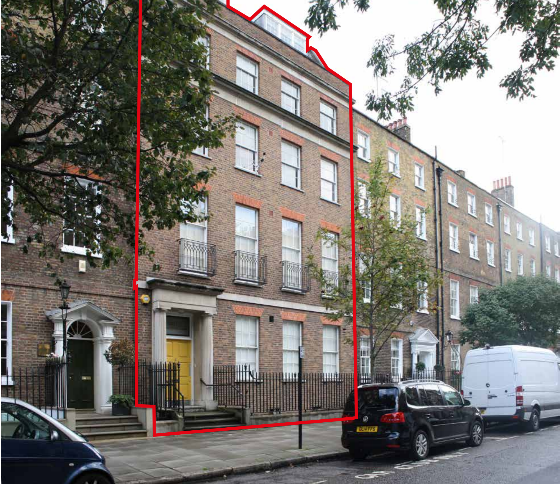
SIDE VIEW FROM JOHN STREET SHOWING MID-TERRACE LISTED FACADE
