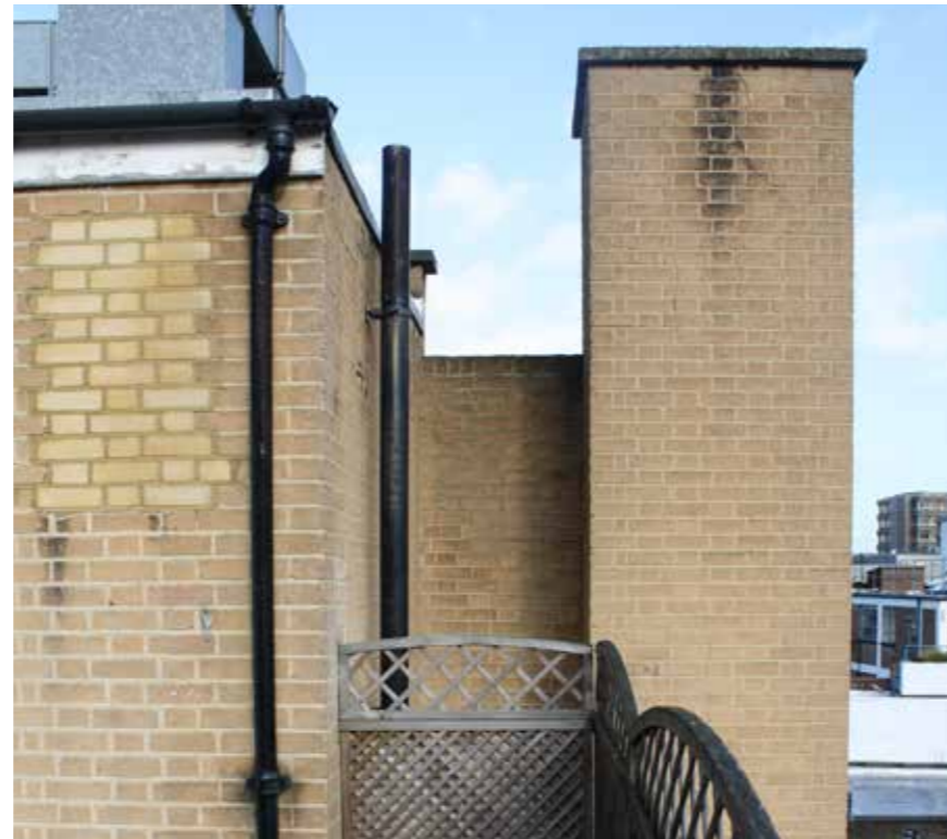
INDUSTRIAL CHIMNEY TO REAR
