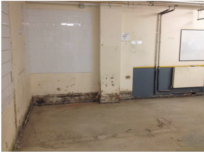
Photograph 4: Training centre (lower ground floor)
