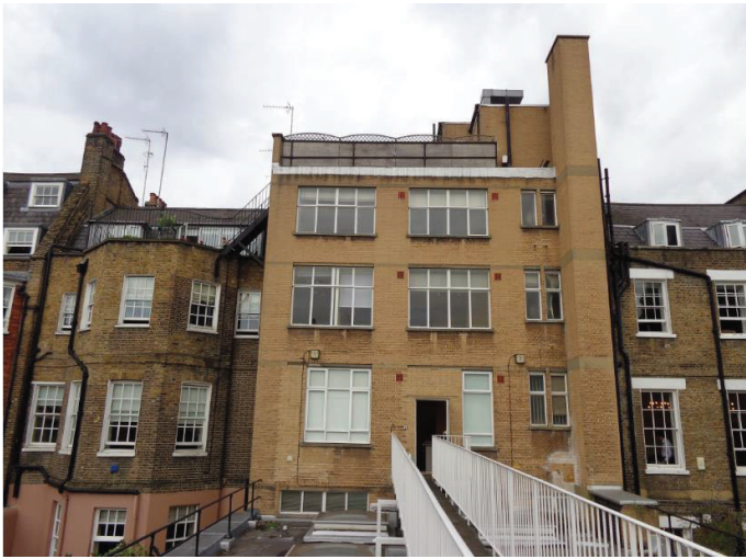
Photograph 7: Small ancillary offices (second floor)
