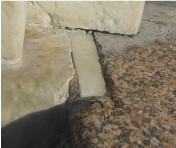
Failing pointing on previous repairs.
