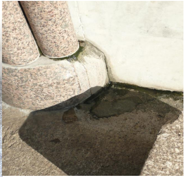
Active leaks though masonry on west side.
