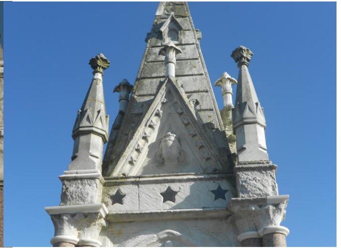
Decayed marbles on frieze of west elevation.
