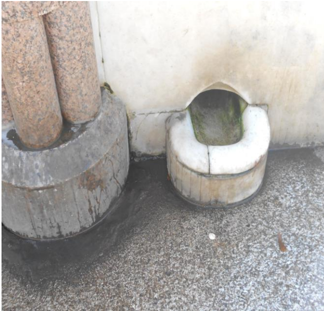
Leaks though masonry joints on north side.
