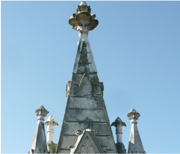
Marble spire requiring cleaning and repair.
