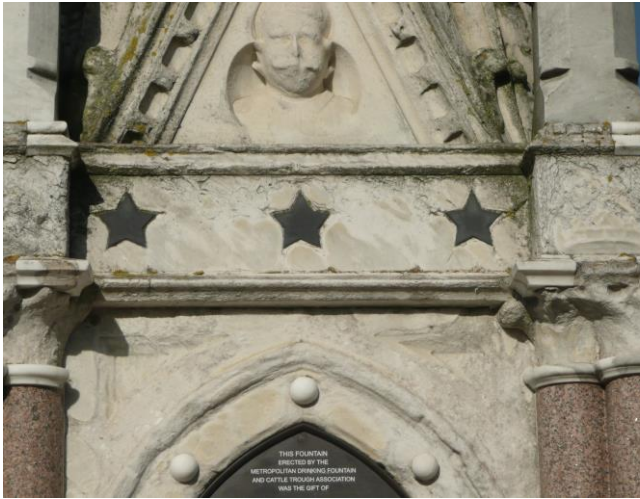
Decaying marbles on the south elevation.
