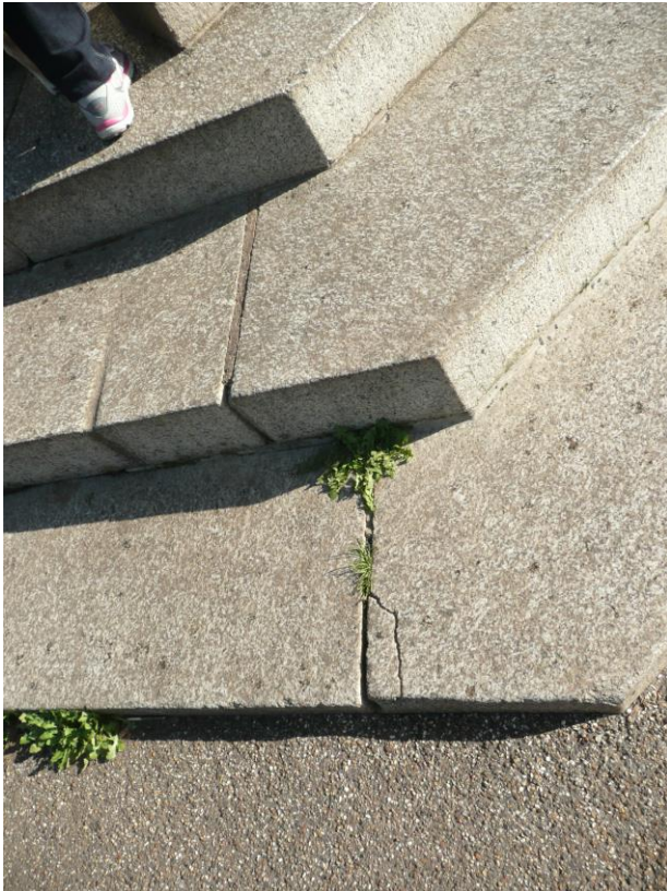
Open joints and crack on steps
