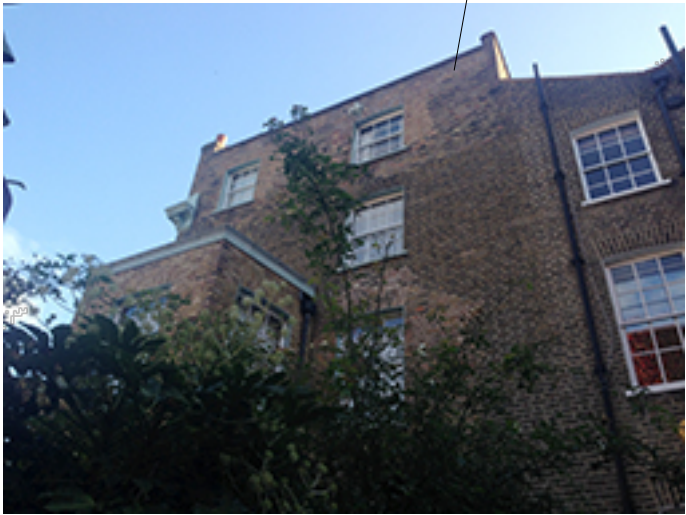
2. View to No.39 Rear Elevation
