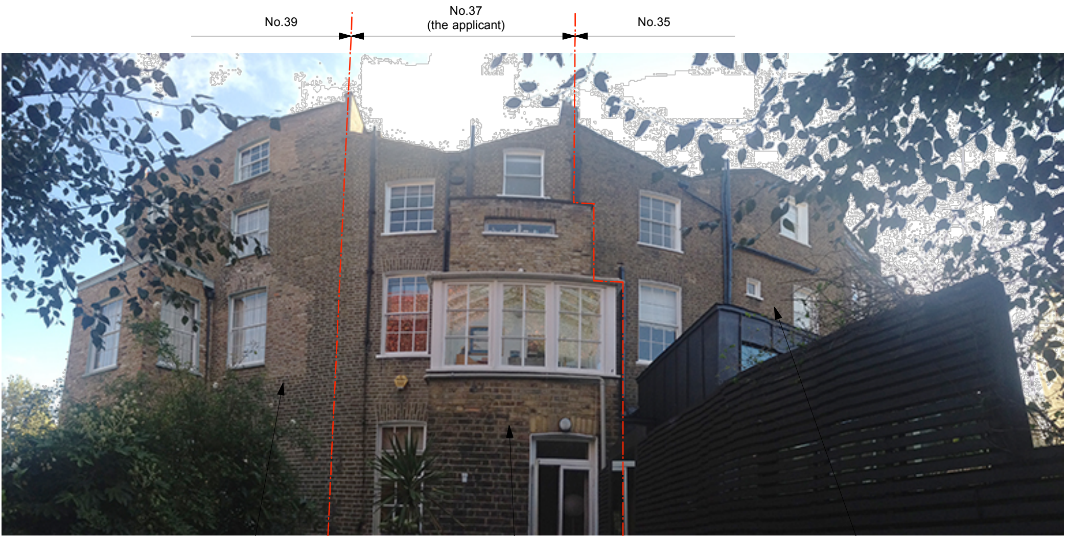
1. Panorama view of Rear Elevations
