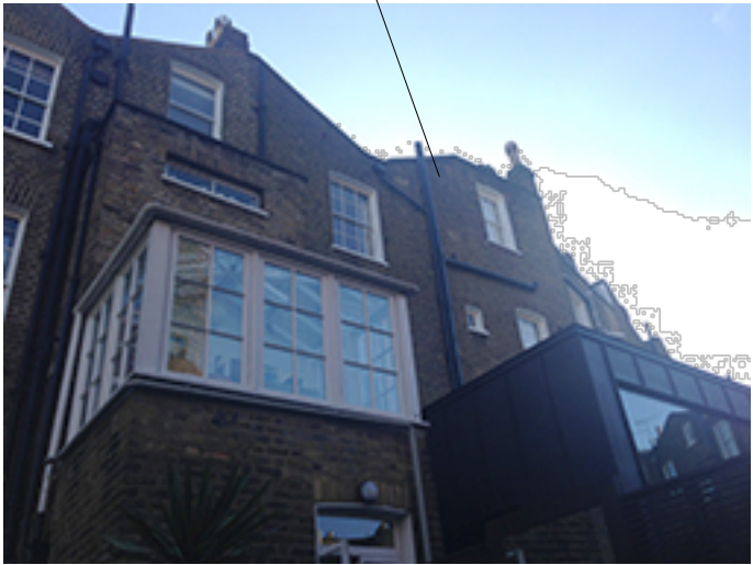
4. View to No.35 Rear Elevation
