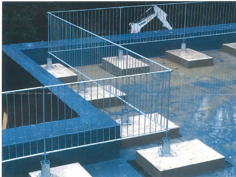
Photo 2: Installed Metal Barrier – Close up Shot
