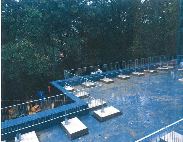
Photo 1: Installed Metal Barrier – Wide Shot
