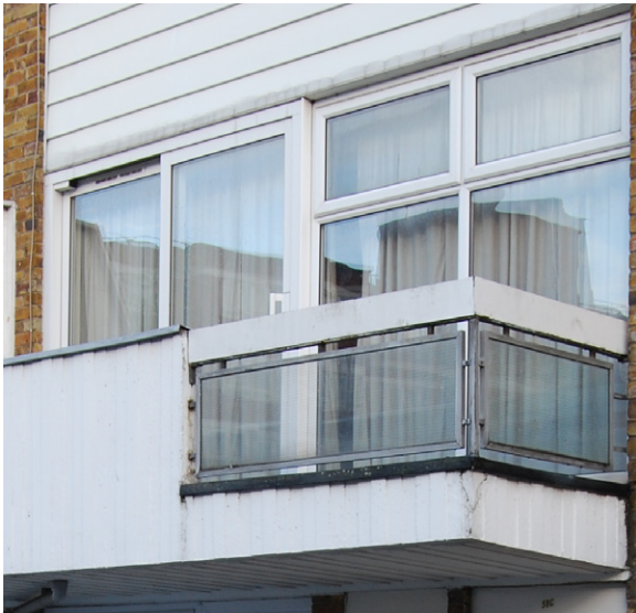
Image 1.4 Existing balcony and spandrel panels
