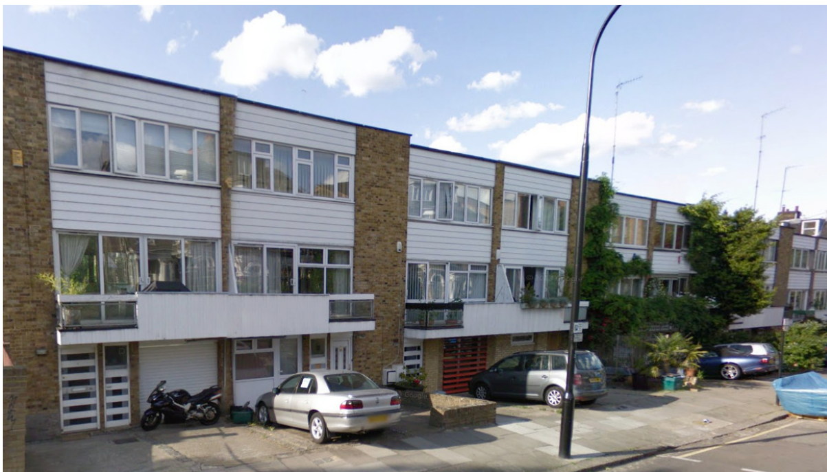
Image 1.1 Street view of terrace houses (Left to right : 58D, 58C, 58B, 58A, 58,56E,56D, 56C,56B King Henry's Road.
