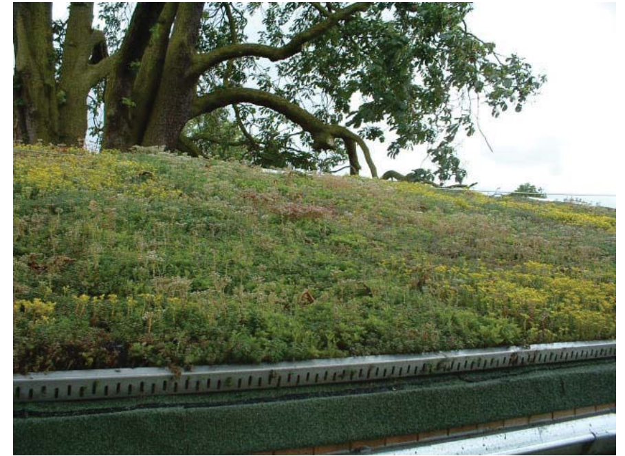
PICTURE OF GREEN ROOF WITH SEDUM BLANKET
