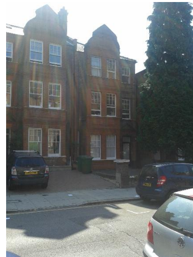
Figs.1&2 Photos of front & rear of No. 67
