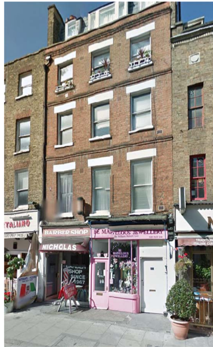
02 EXISTING VIEW - BUILDING SCALE : NTS
