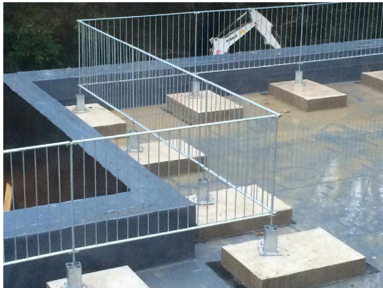
Photo 2: Installed Metal Barrier – Close up Shot
