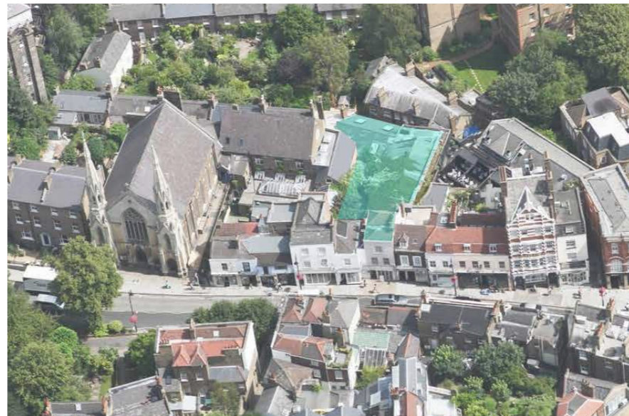
Ariel view of 76 Heath Street from West
