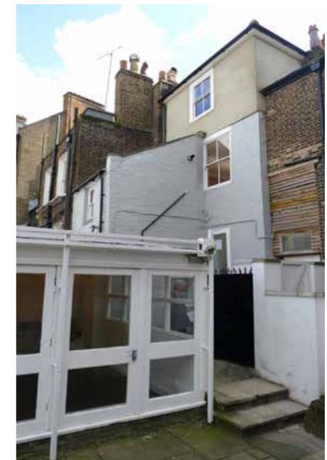
Rear facade of 76 Heath St
