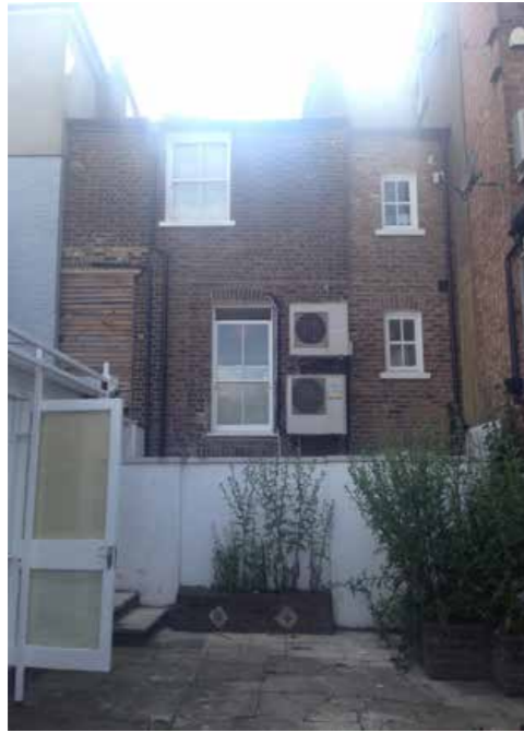
View from courtyard towards Rear facade of 76 Heath St
