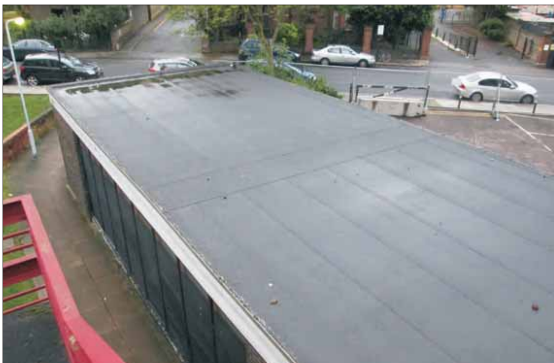
PHOTOGRAPH 4: Roof of Building B2
