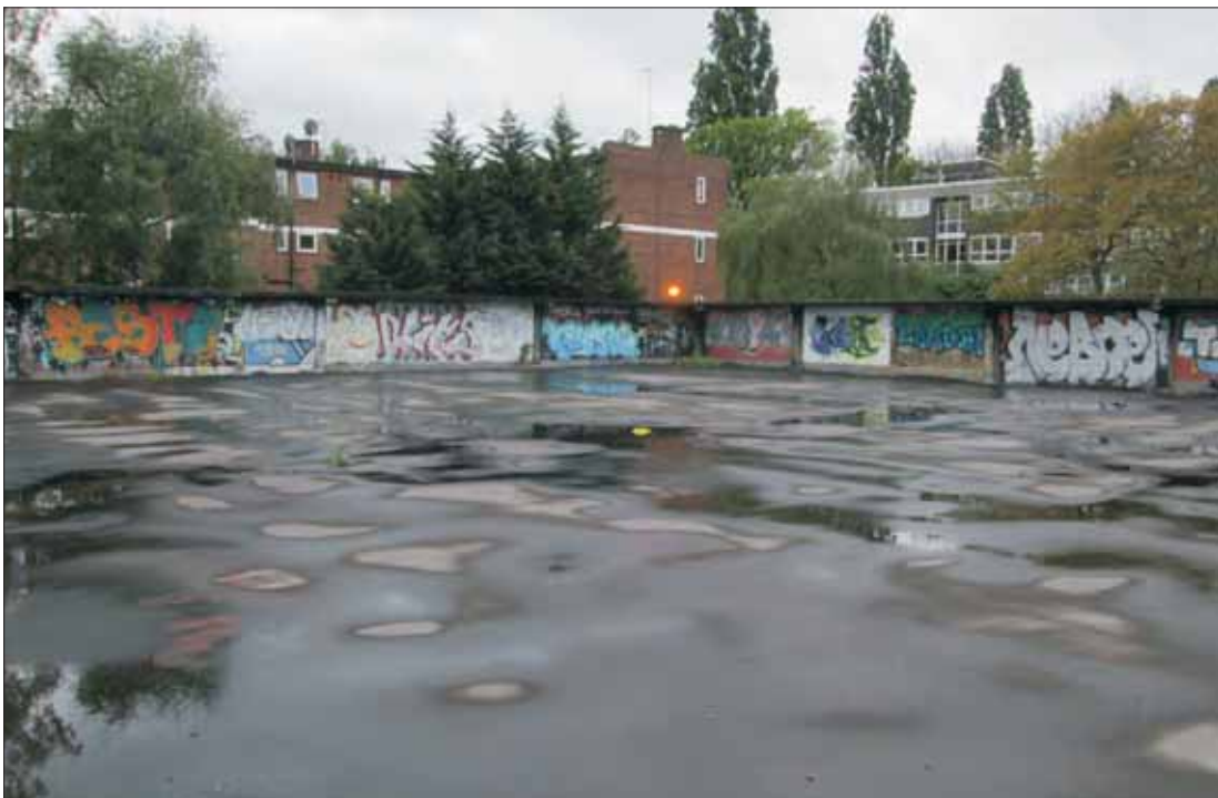
PHOTOGRAPH 2: Roof of Building B1
