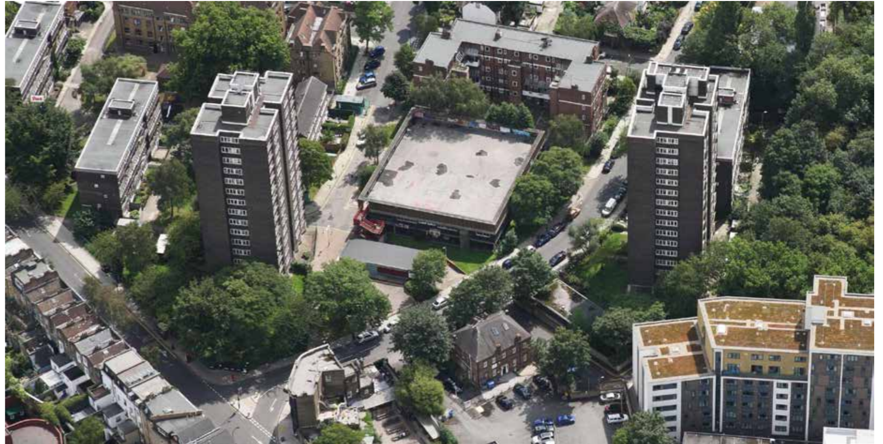
Existing car park and community centre buildings on site
