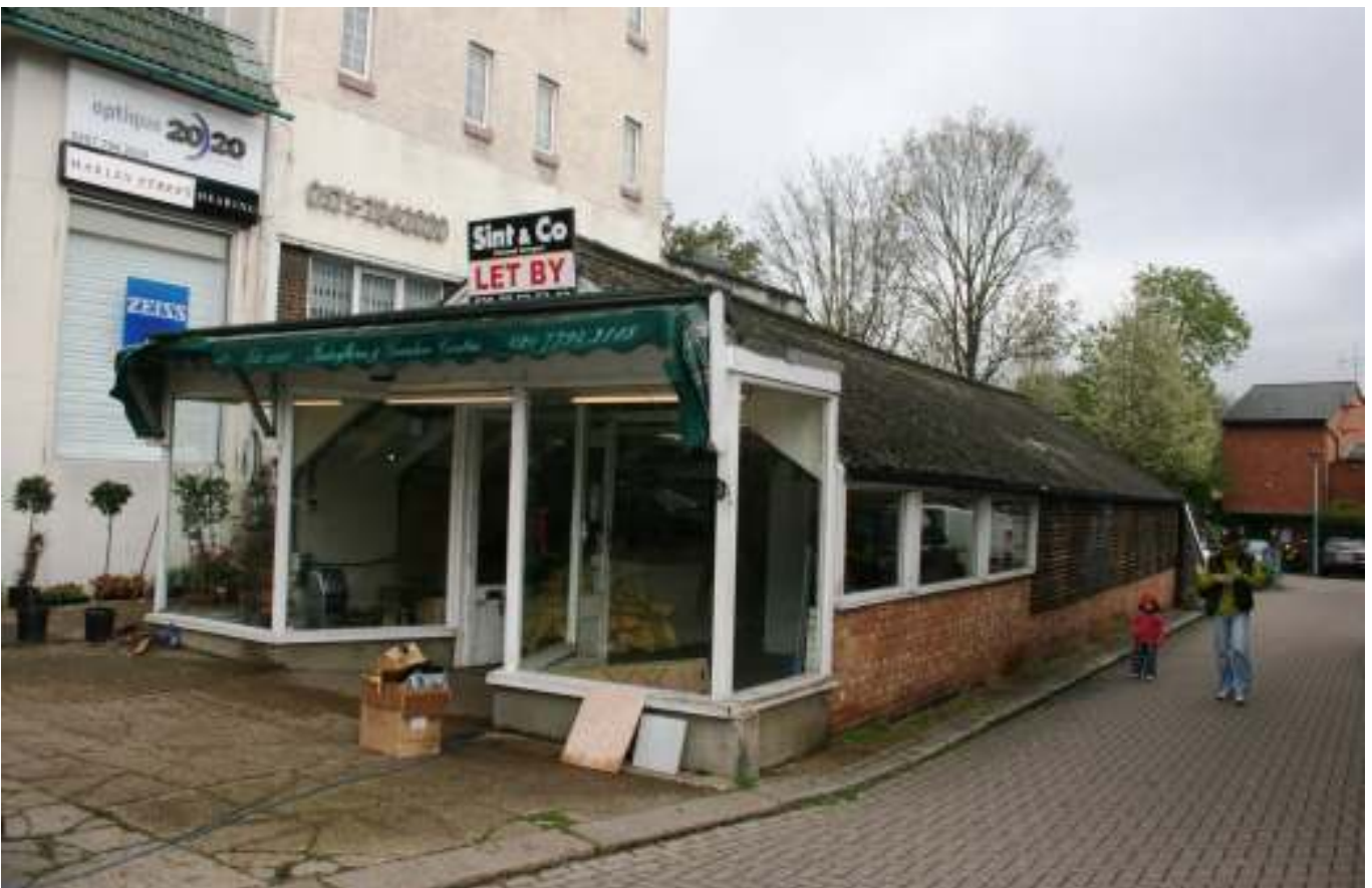
Photo 2 192 Haverstock Hill with shared access to south leading to the Globe Tennis Club to rear. Note 1 Shared access drops 0.6m along side of shop and 1.0m overall from front to rear
