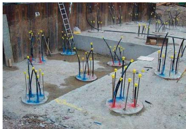
Energy piles in place
