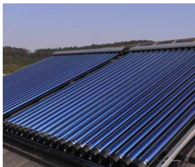
Evacuated Shell and Tube Solar Thermal Panel
