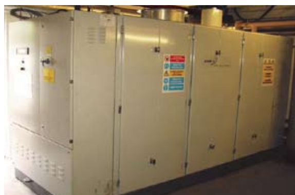
Ener-G 150kW CHP. The development will not have enough hours of demand to run a CHP system efficiently
