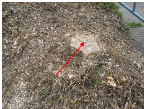
Decay in stump in tree pit north
