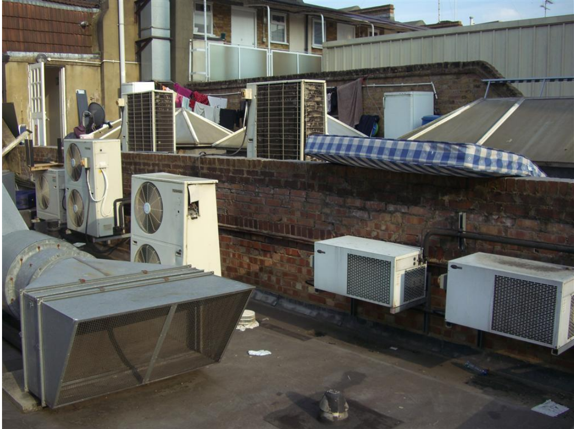
Refrigeration condensers in the vicinity of the fresh air inlet. In the background an access balcony to flats can be seen.
