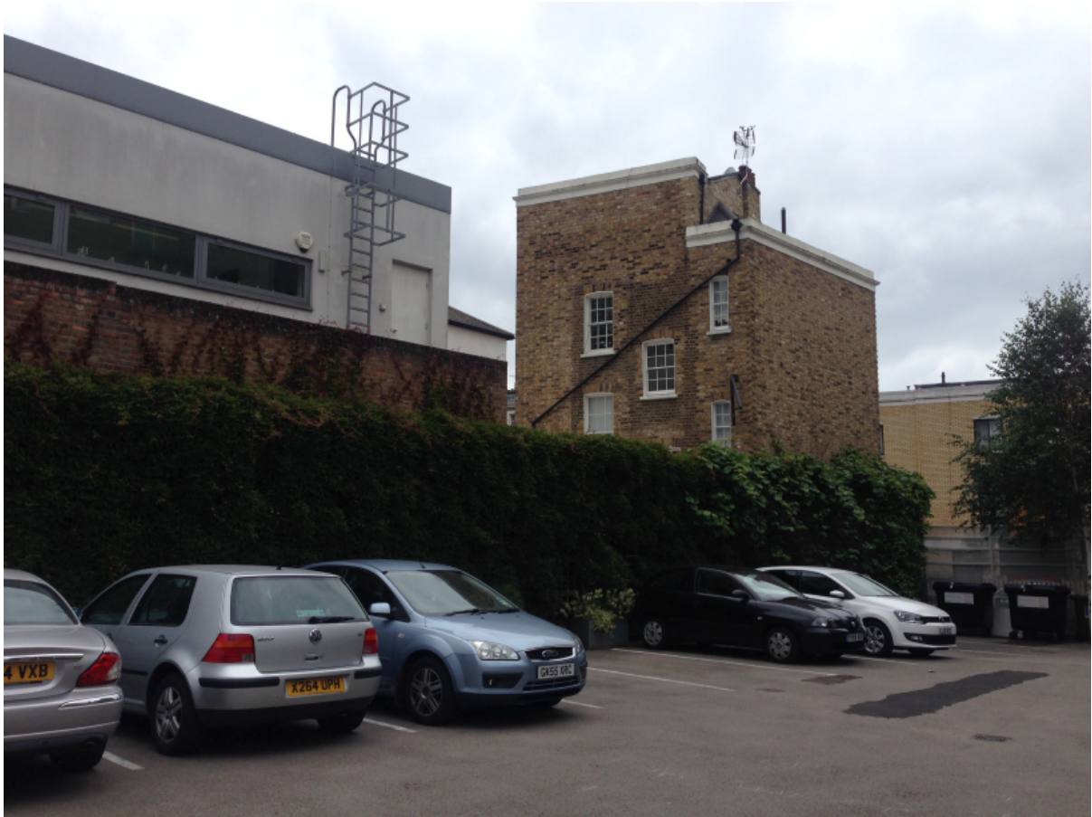
Photo 3. Rear of No.33 Inverness Street and No.35 (Clearwater Yard)
