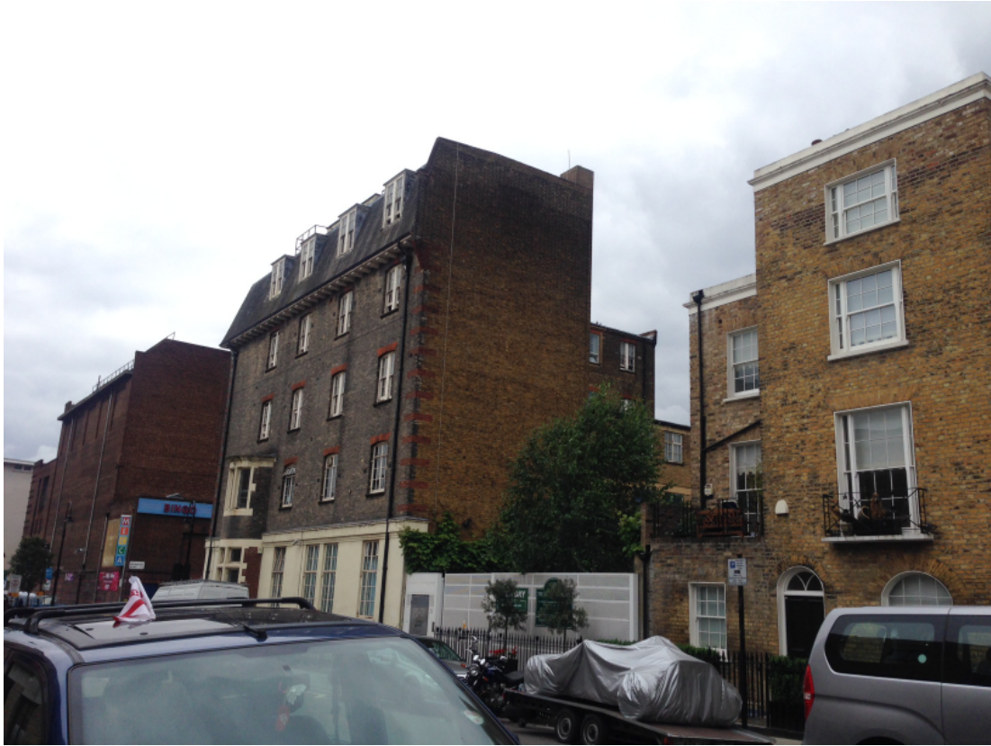
Photo 5. View from west of Inverness Street
