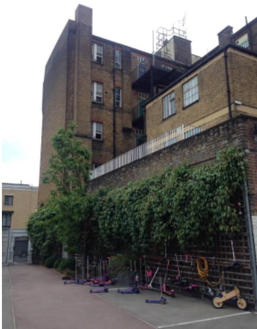
Photo 4. Rear of Camden House
