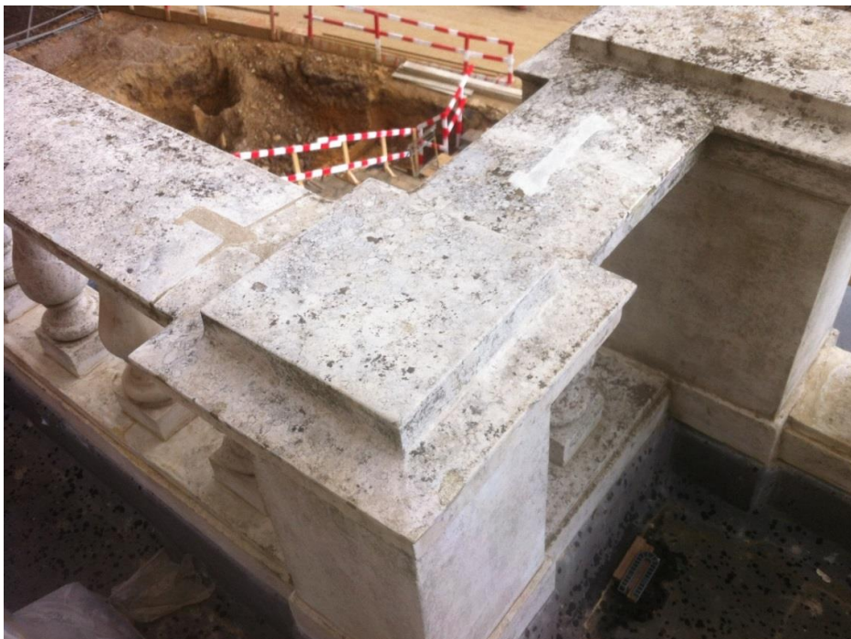
4. Existing stone balustrade to rear second floor terrace.
