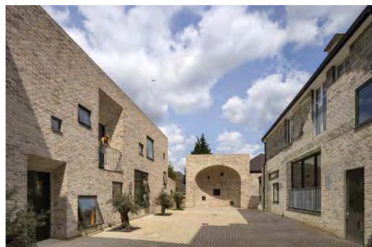
Recently completed PBA building showing possible materiality
