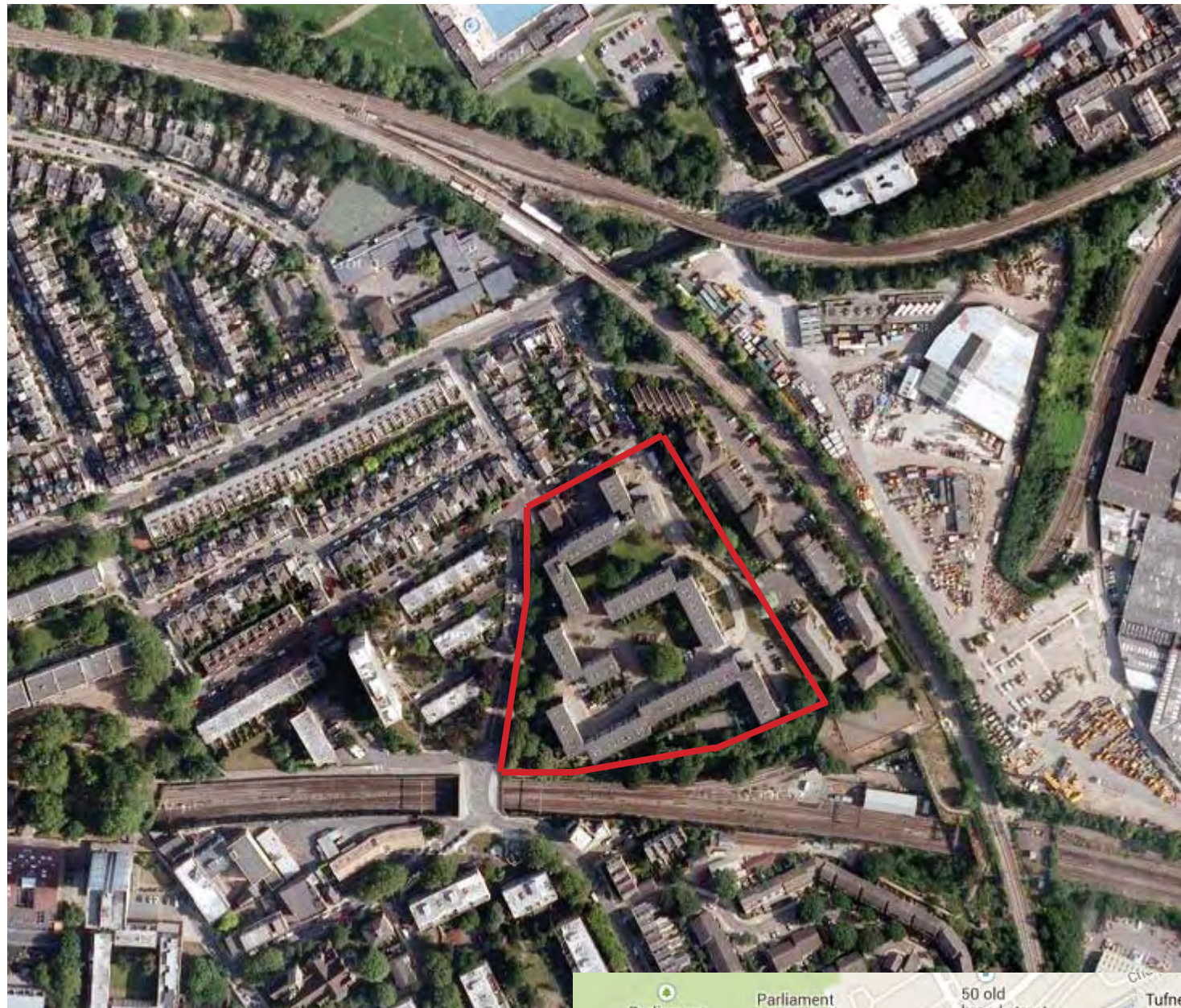
Aerial View of Gospel Oak - Kiln Place Estate shown in red boundary
