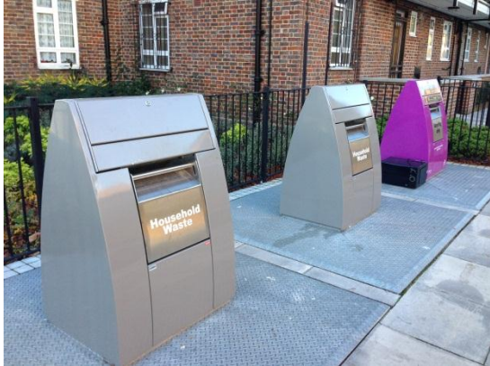
Photo 1: External surface view of the SULO underground waste containers.
