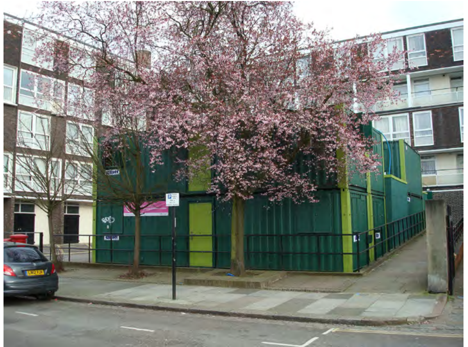
Site Portacabins in the north of Kiln Place
