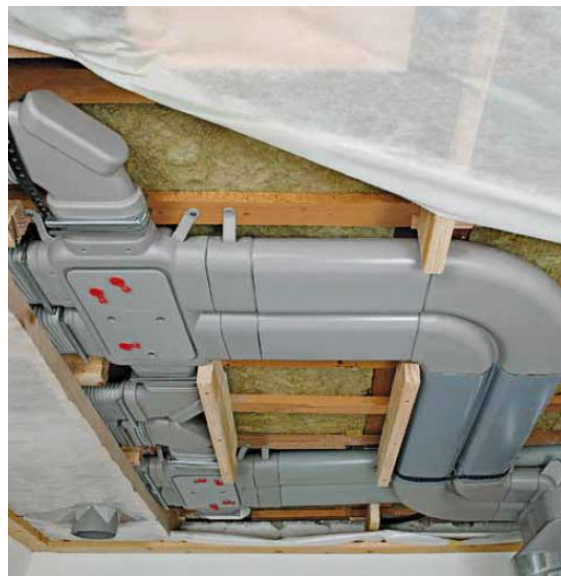
Figure 8: Concealed ductwork routing (a); MVHR application (b)
