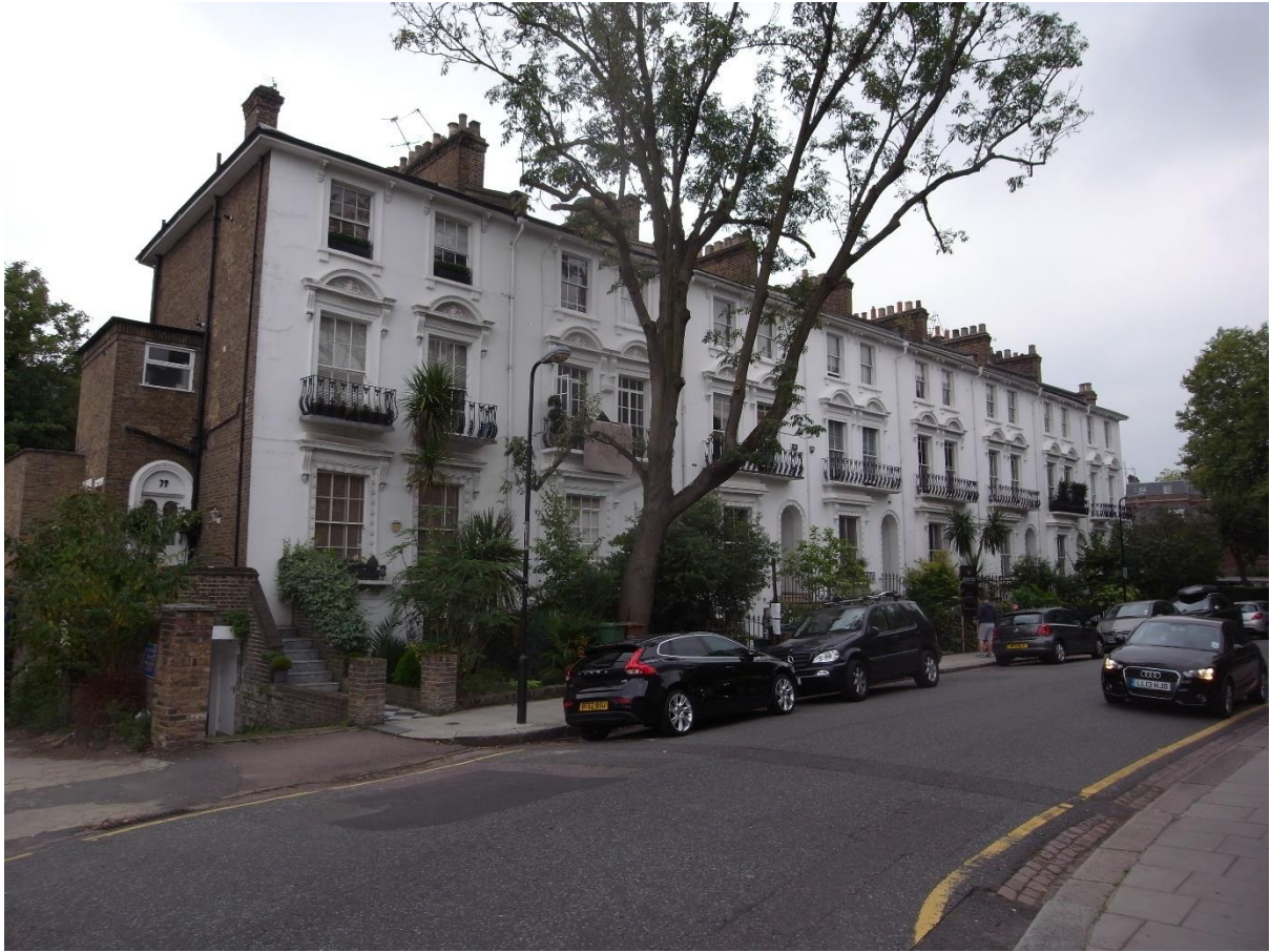
Front of listed terrace (No. 81 is second left behind tree)
