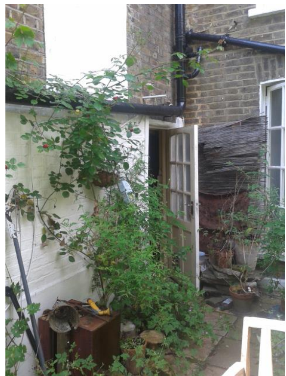
View towards back door from garden.
