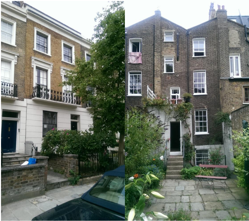
Front Façade and Roof, rear Front Façade and Roof
